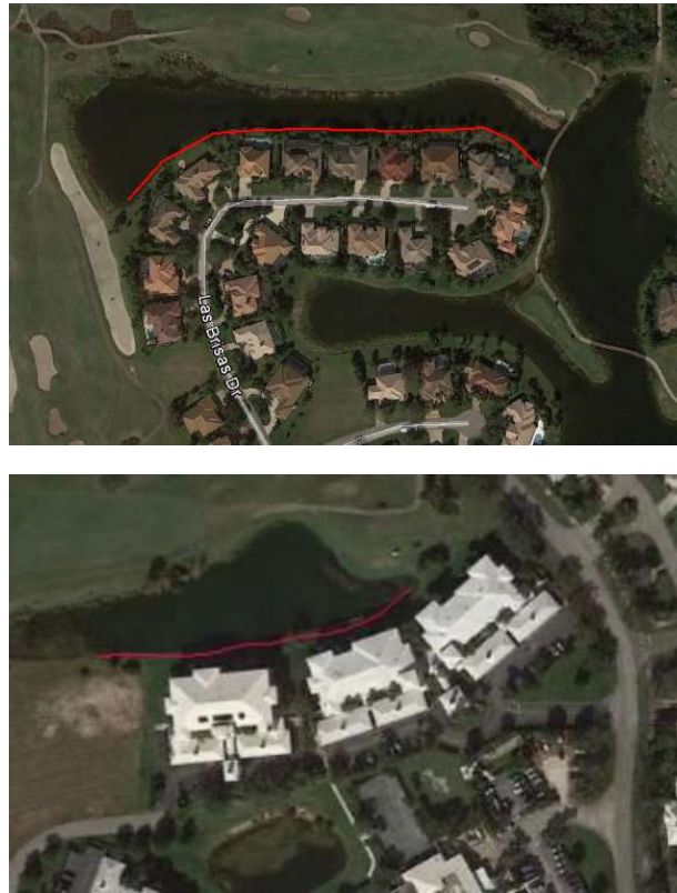
Photo 8.1 and 8.2– Bank erosion area encroaching onto properties
