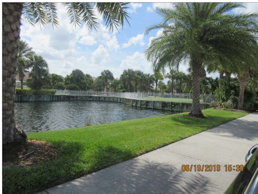
Photo 18.11 – Overview of wood retaining wall
