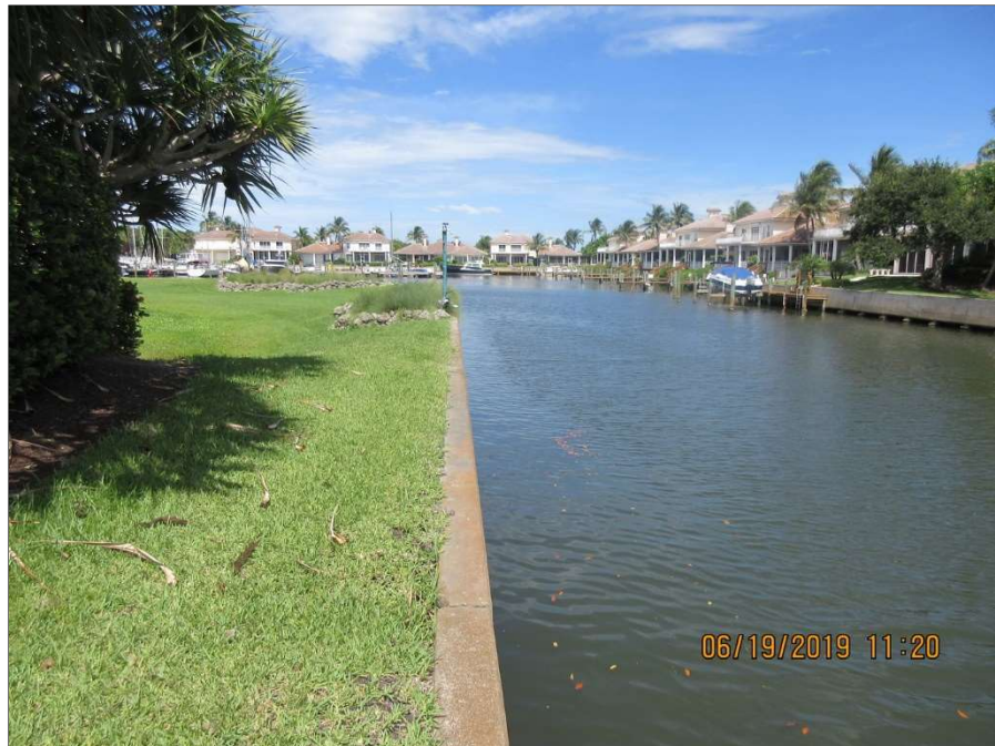
Photo 18.4 – Overview of Retaining wall Span #1
