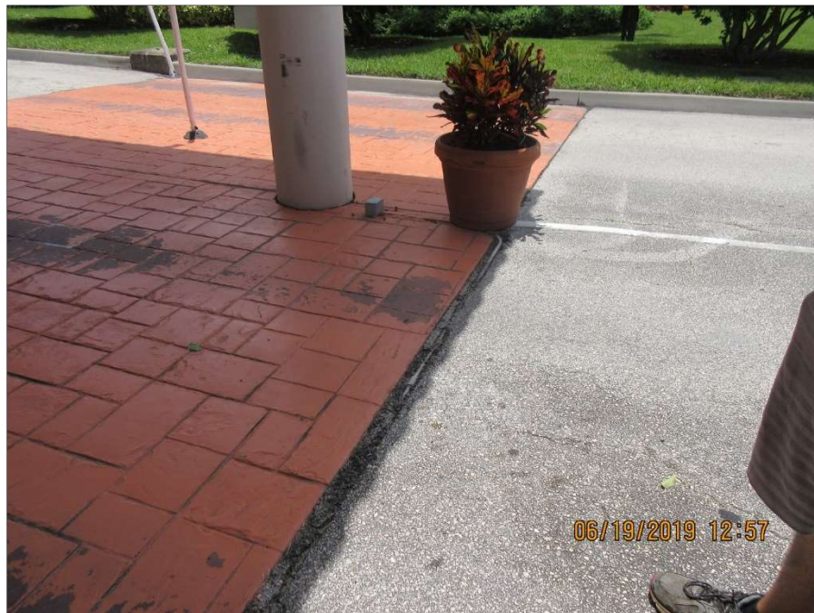
Photo 17.4 – Exposed PVC conduit casing at Guard House #1
