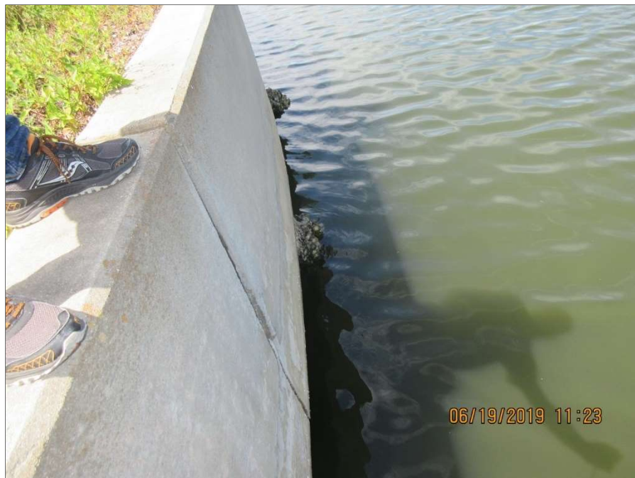
Photo 18.6 –Overview of the water-side edge of Retaining wall Span #1
