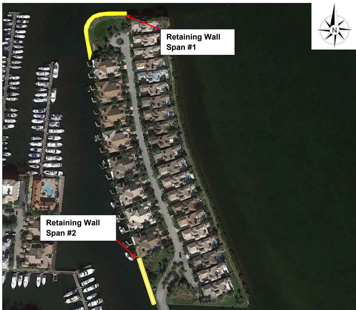
Figure 18.1 – Aerial Photograph of Retaining Wall Spans #1 and #2 (Source: Google Earth)
