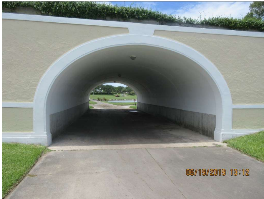
Photo 19.11 – Overview of Tunnel #3
