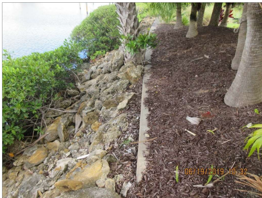
Photo 18.9—Rock revetment covered the water-side; landscaping covered the land-side of Retaining wall Span #2
