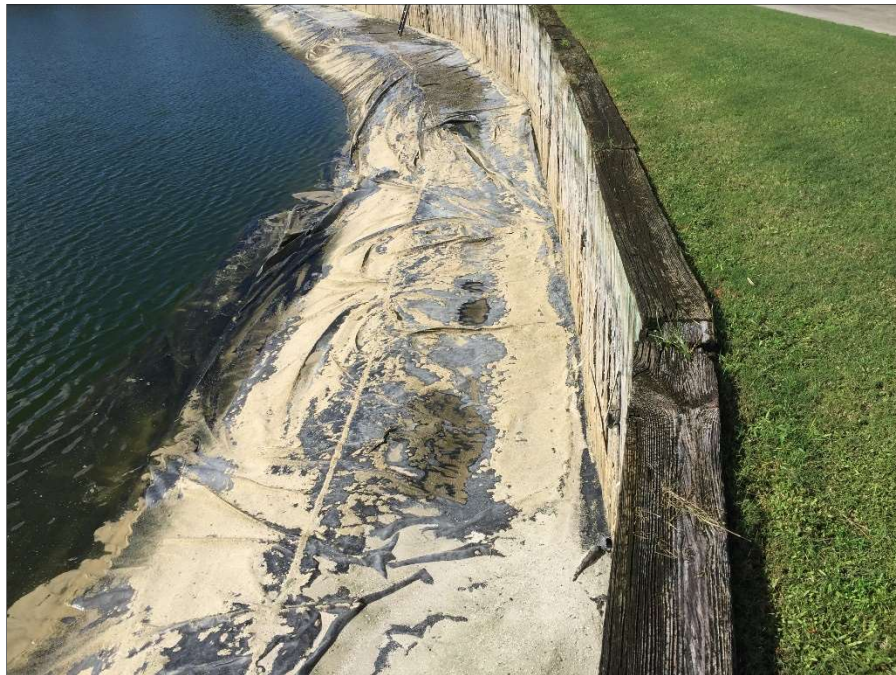
Photo 18.21 – Pond liner in the recycled water reservoir with Retaining wall Span #4
