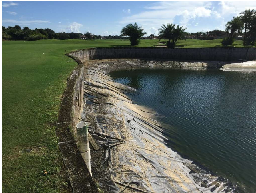
Photo 18.20 –Pond liner in the recycled water reservoir with Retaining wall Span #4
