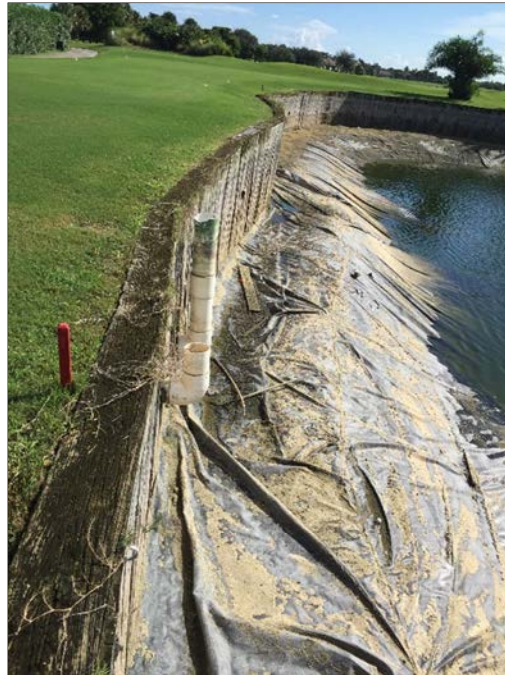
Photo 18.22 – Pond liner in the recycled water reservoir with Retaining wall Span #4
