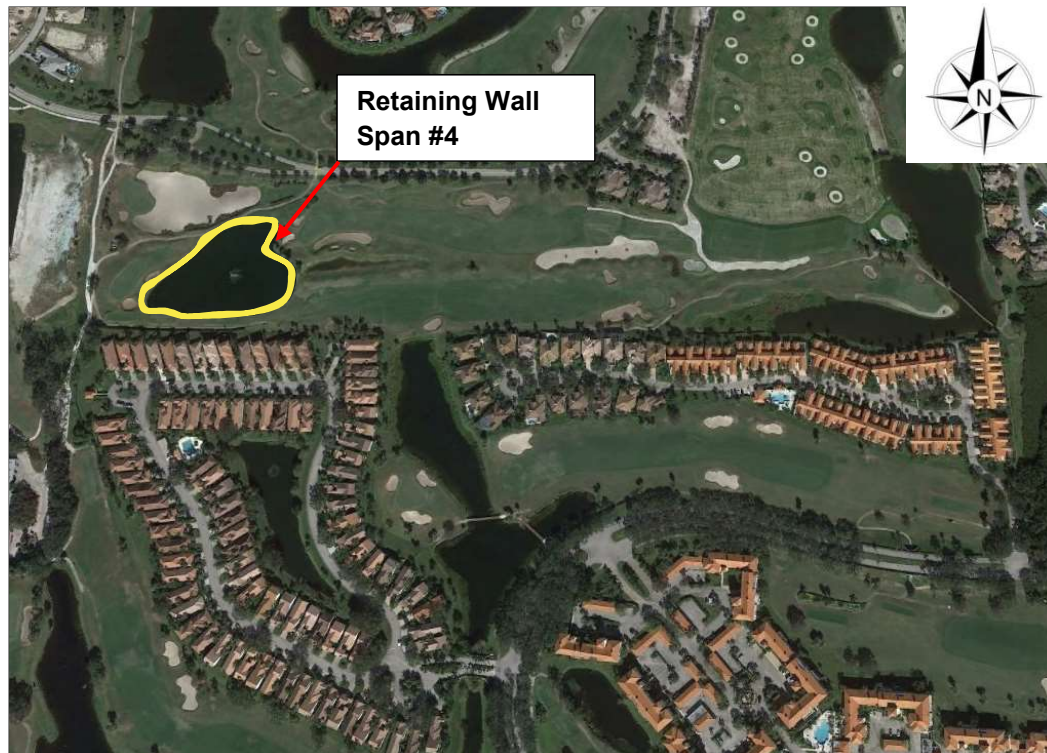
Figure 18.3 – Aerial Photograph of Retaining Wall Spans #4 (Source: Google Earth)
