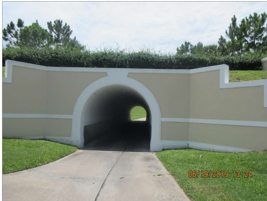
Photo 19.15 – Overview of Tunnel #4
