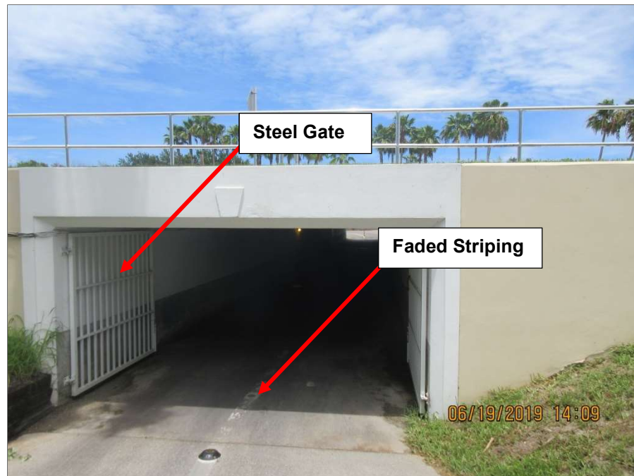
Photo 19.1 –Steel Gate at entry of Tunnel #1. Note faded striping.
