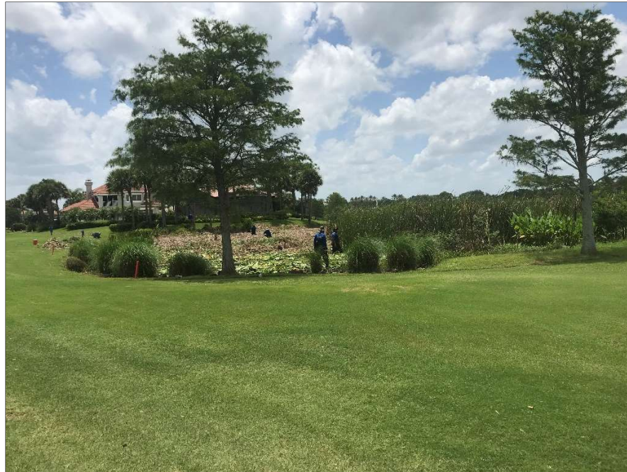
Photo 8.9 – Maintenance crew removing cattail from littoral zone
