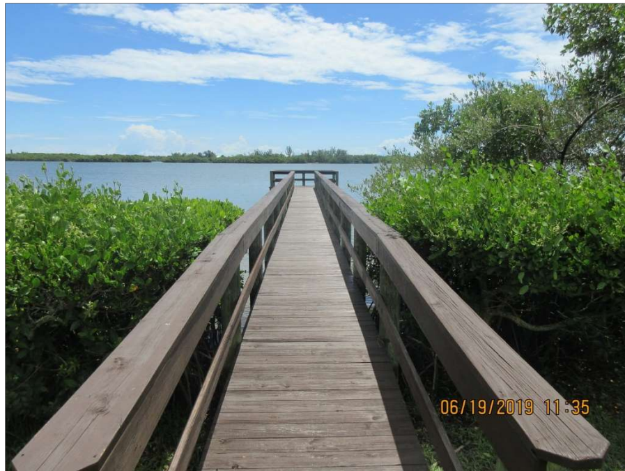
Photo 20.1 –Overview of River Village Pier
