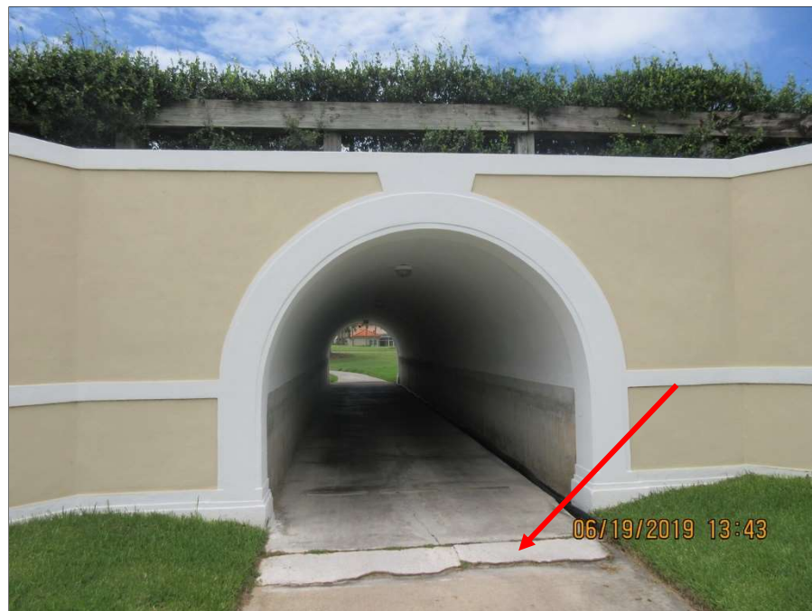
Photo 19.8 – Post-modified topping slab at Tunnel #2
