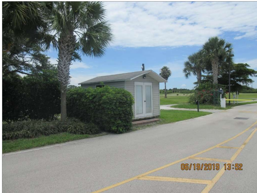
Photo 20.5 – Overview of Via Marbella Guard Shack
