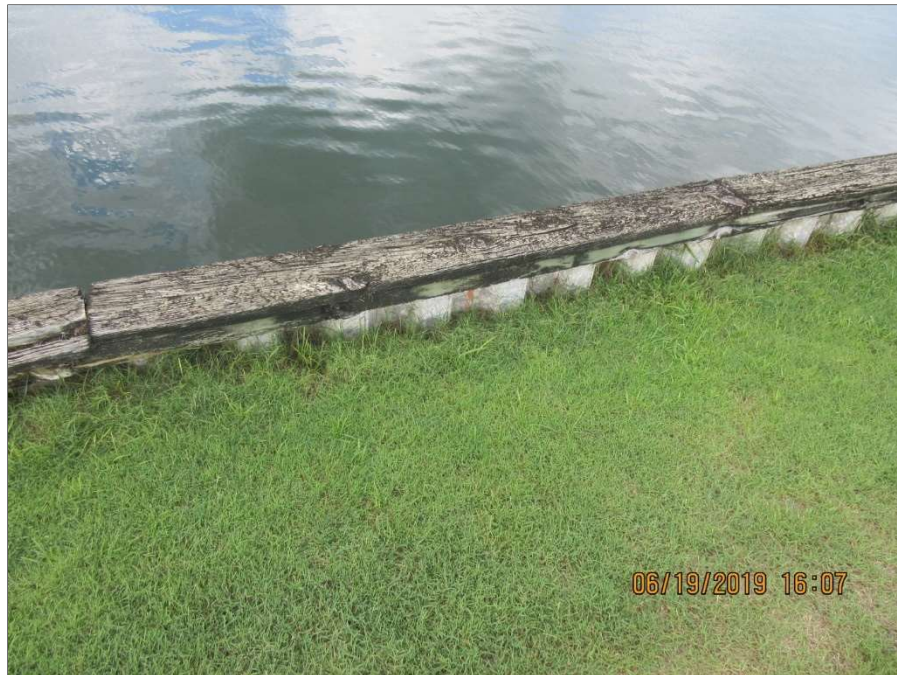
Photo 18.18 –Exposed portion of landside of Retaining wall Span #4
