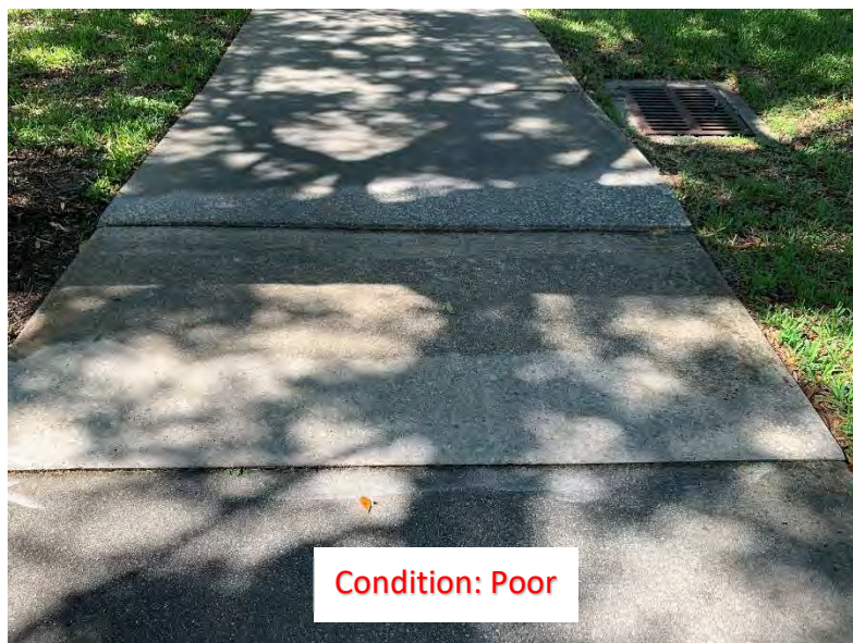
(238) Elevated Corner/Slab
