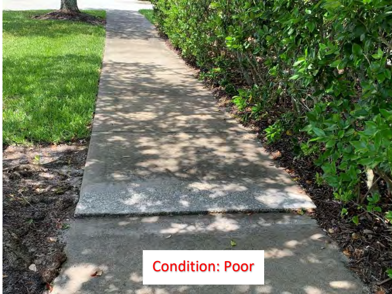
(275) Elevated Corner/Slab
