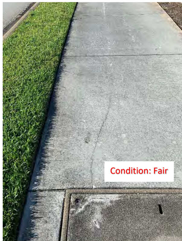
(177) Center Crack
