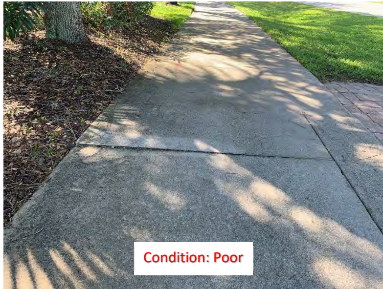
(210) Elevated Corner/Slab
