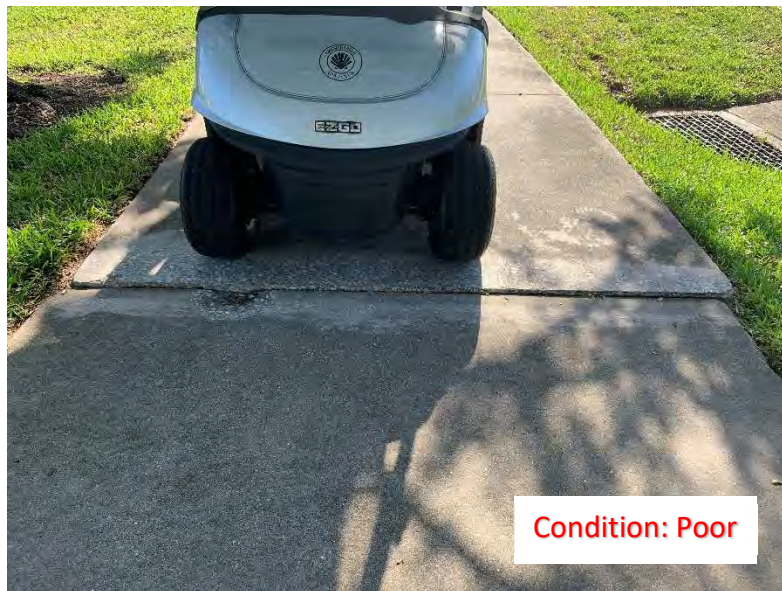
(200) Elevated Corner/Slab
