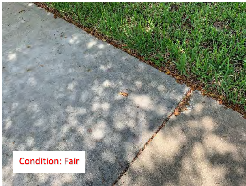
(258) Corner Cracks (2)
