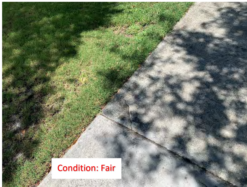
(304) Corner Crack
