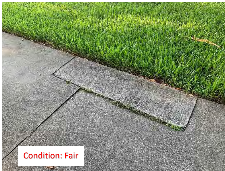
(149) Elevated Corner/Slab (2)
