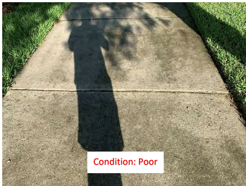
(159) Elevated Corner/Slab (1)
