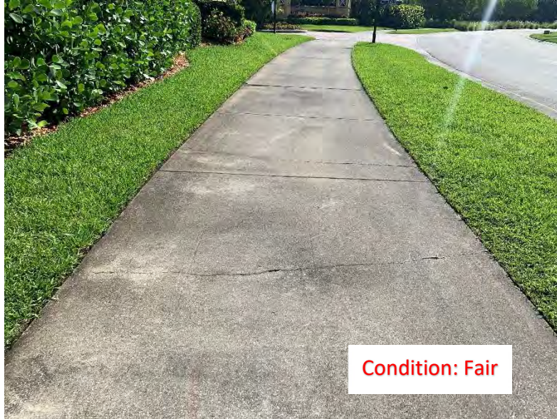
(225) Center Cracks (1)
