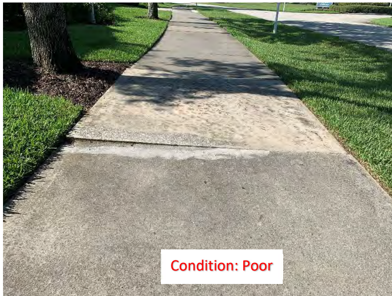
(217) Elevated Corner/Slab (2)
