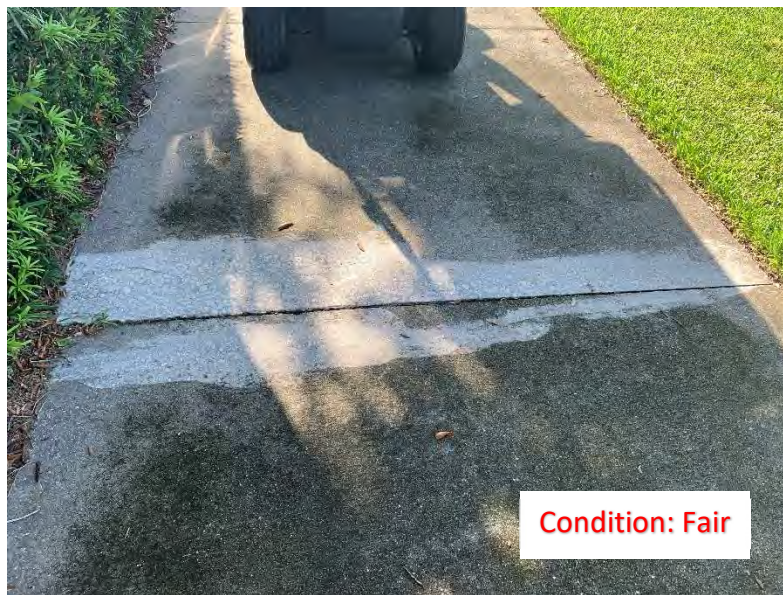
(193) Elevated Corner/Slab
