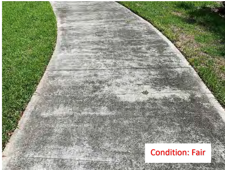
(259) Center Crack
