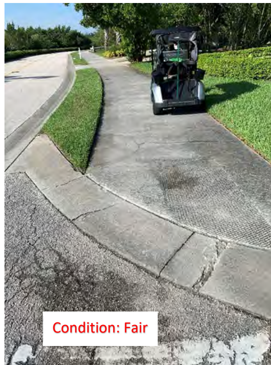
(187) Center Cracks (1)
