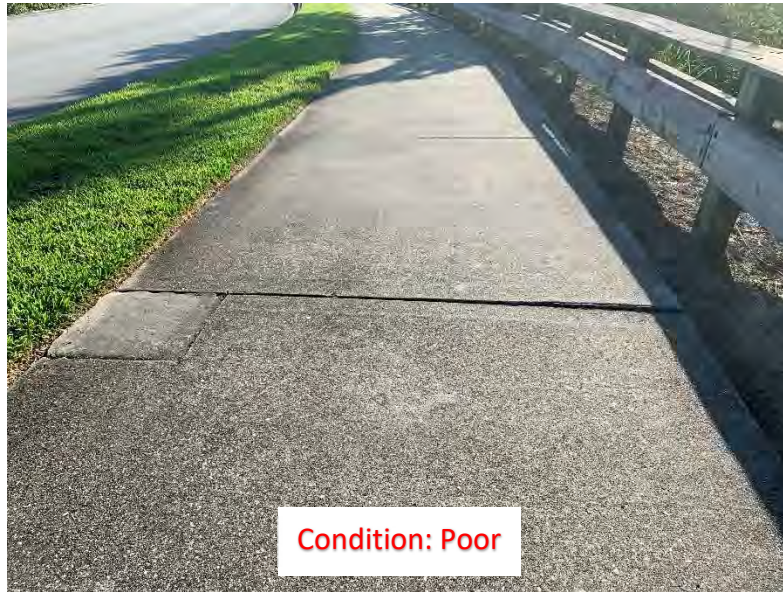
(160) Elevated Corner/Slab (2)
