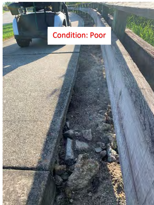
(161) Sidewalk Undermining
