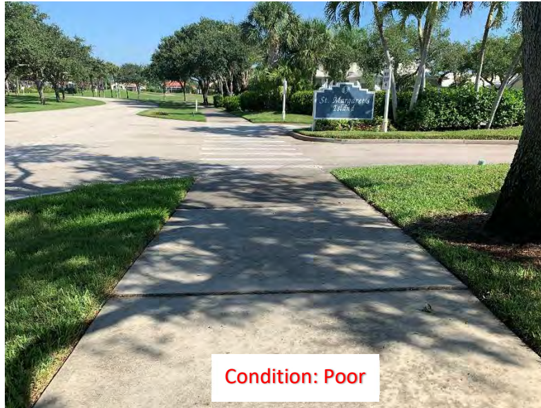
(222) Elevated Corner/Slab (1)
