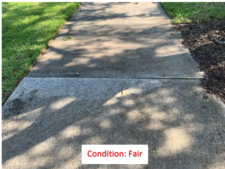
(219) Elevated Corner/Slab (2)
