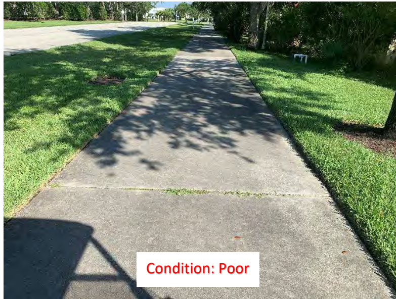
(206) Elevated Corner/Slab
