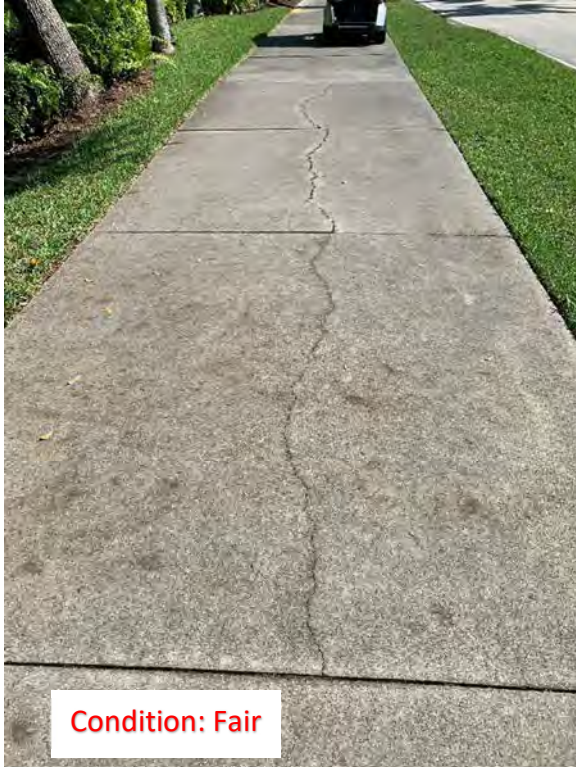
(241) Center Cracks (4)
