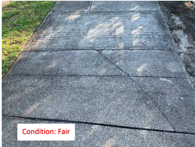
(164) Center Crack
