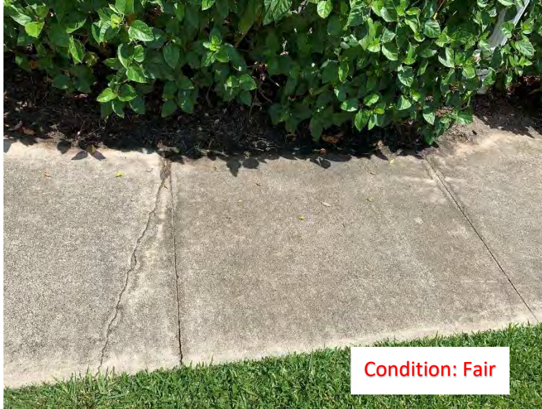
(264) Center Cracks (1)
