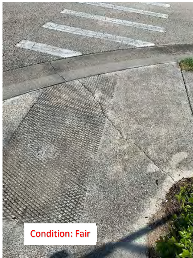
(184) Center Crack
