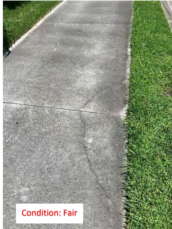
(287) Corner Cracks
