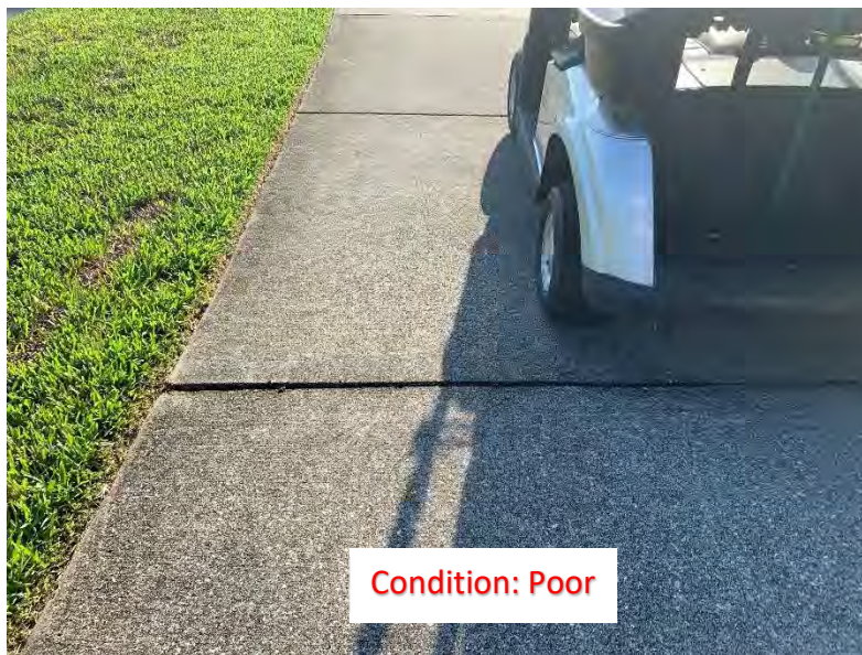
(160) Elevated Corner/Slab (1)
