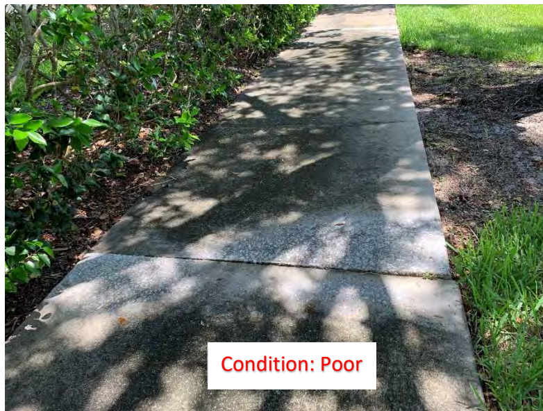
(278) Elevated Corner/Slab
