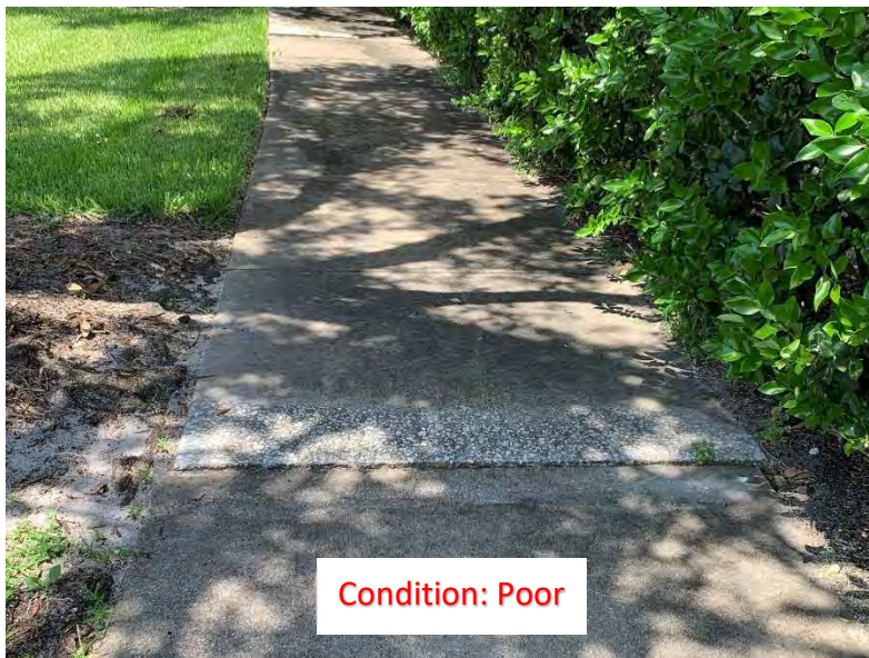
(276) Elevated Corner/Slab
