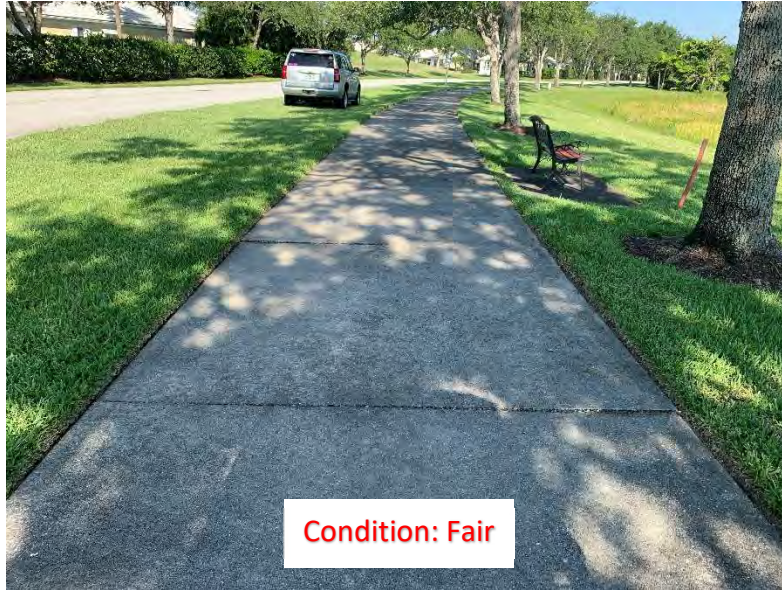
(202) Elevated Corner/Slab (2)
