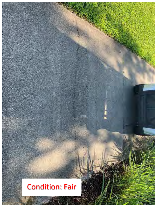
(169) Center Crack
