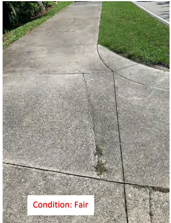
(241) Center Cracks (2)
