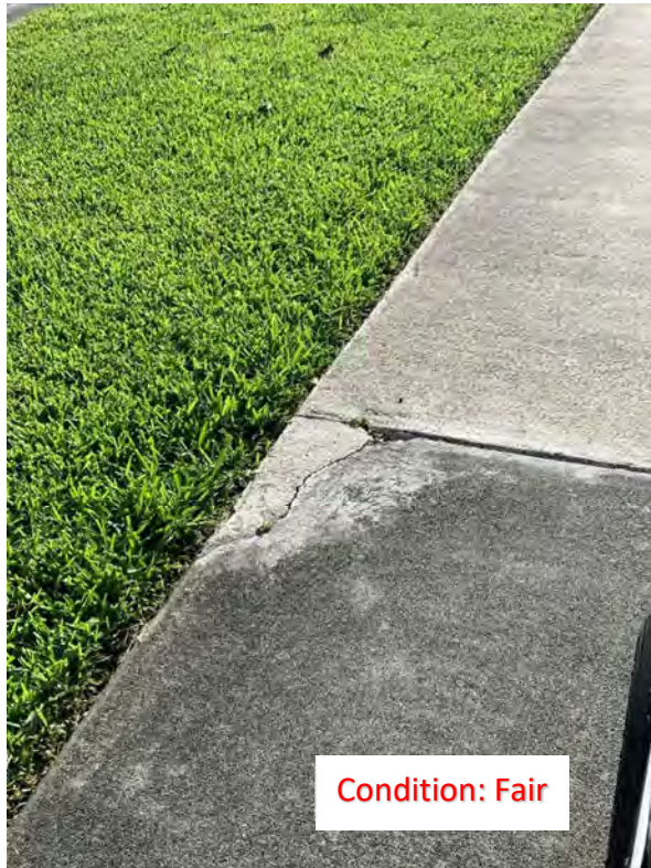
(170) Corner Crack
