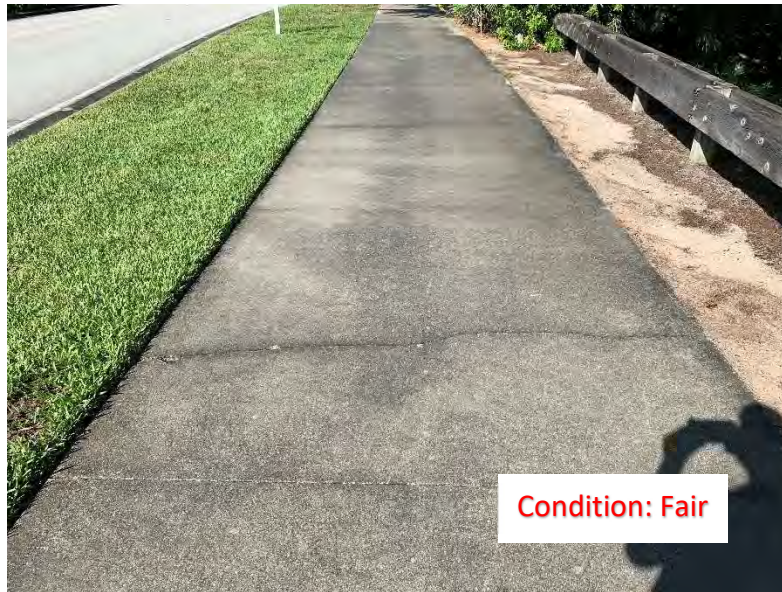
(199) Center Crack
