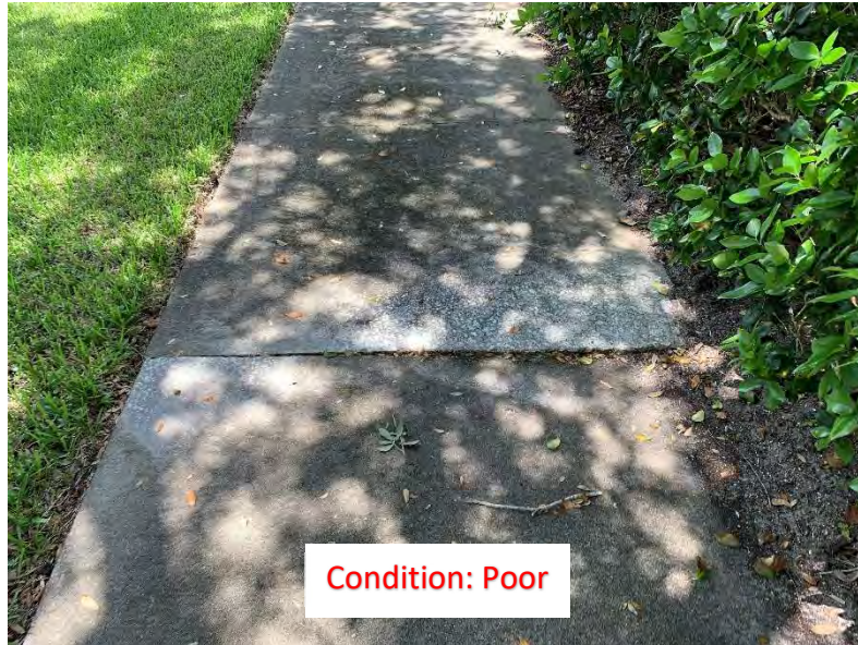
(281) Elevated Corner/Slab
