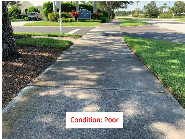
(221) Elevated Corner/Slab (1)
