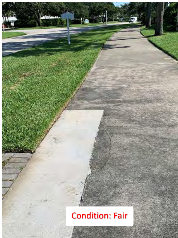
(215) Center Crack
