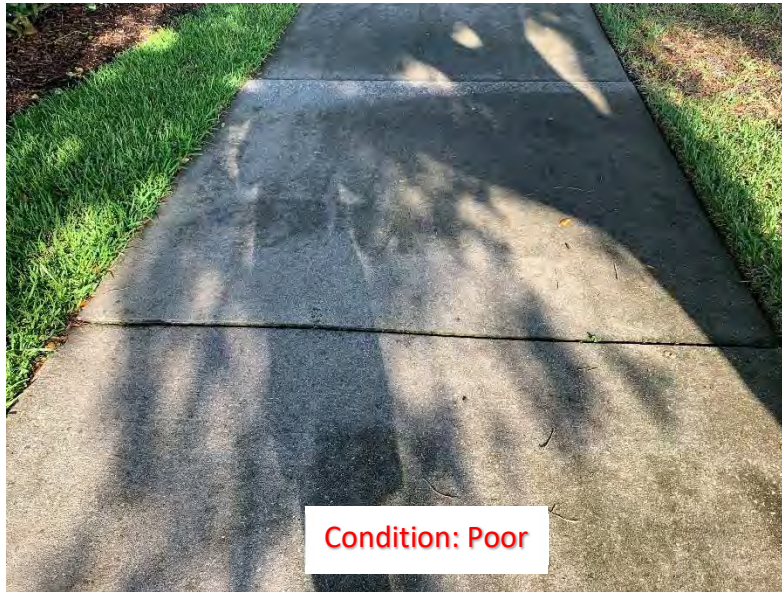
(159) Elevated Corner/Slab (2)
