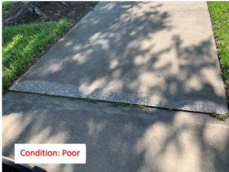
(201) Elevated Corner/Slab
