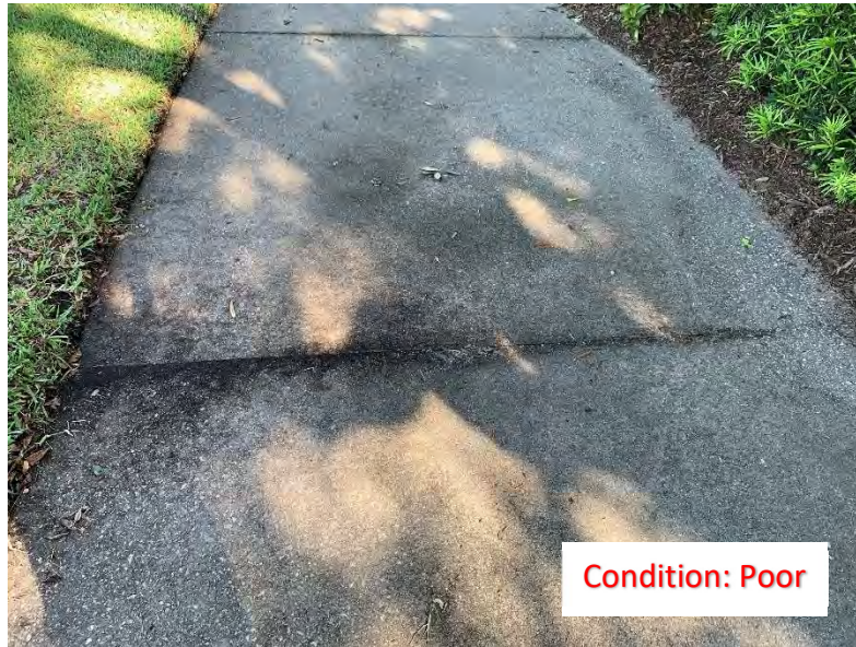
(195) Elevated Corner/Slab (1)
