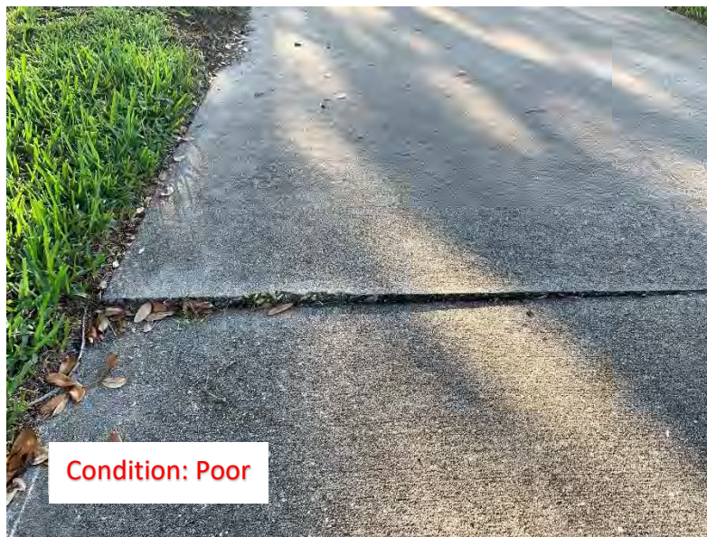
(149) Elevated Corner/Slab (4)
