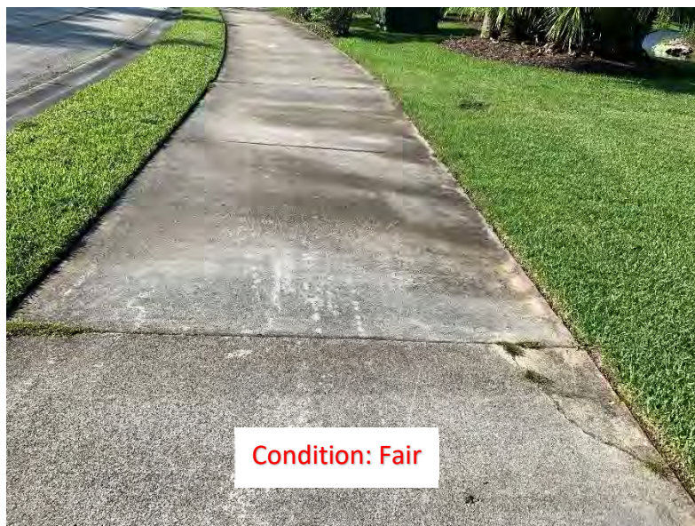
(180) Cracked Corner
