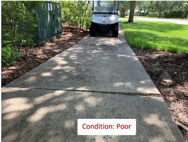
(273) Elevated Corner/Slab
