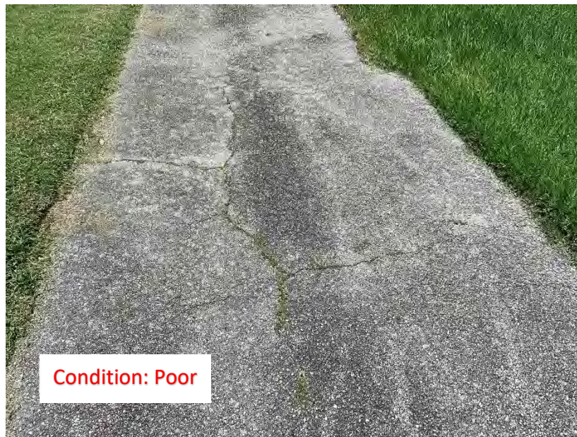
(1) Sidewalk Cracks (2)
