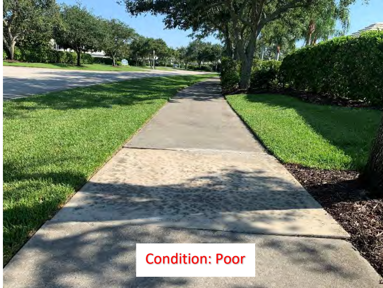
(217) Elevated Corner/Slab (1)
