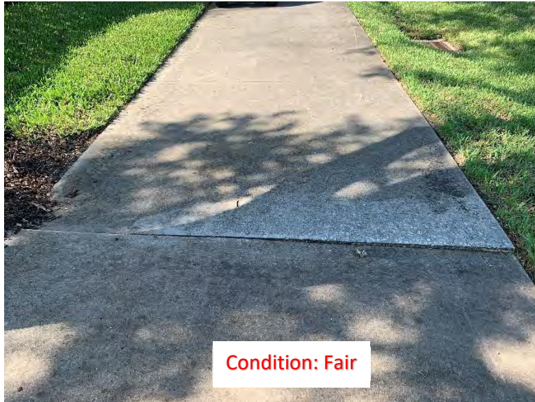
(220) Elevated Corner/Slab (1)
