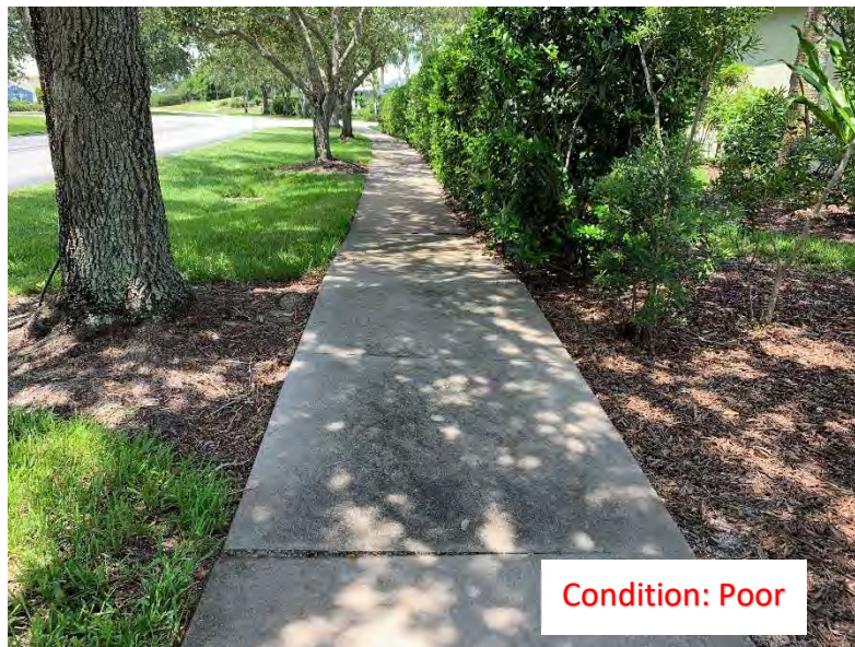
(272) Elevated Corner/Slab
