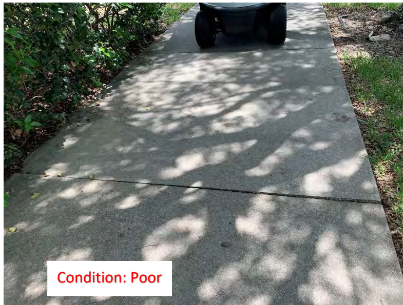
(267) Elevated Corner/Slab (3)
