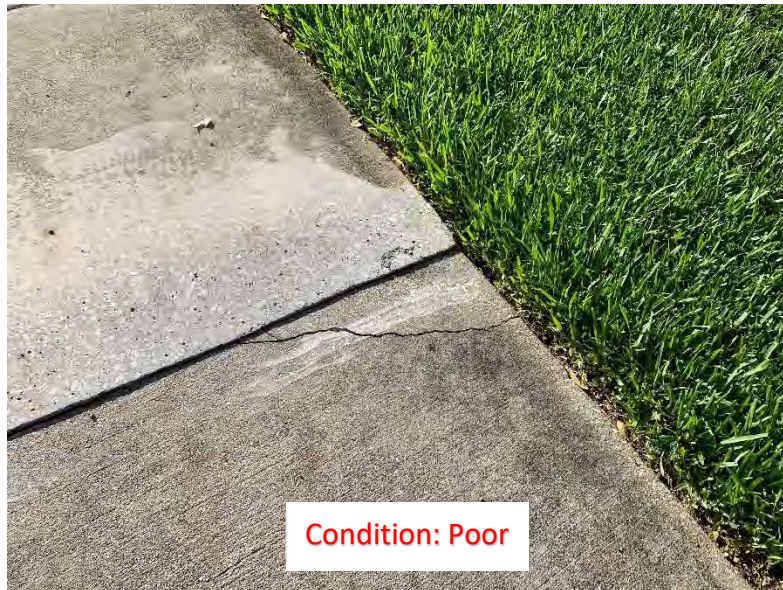
(152) Center Cracks and Corner Crack (1)
