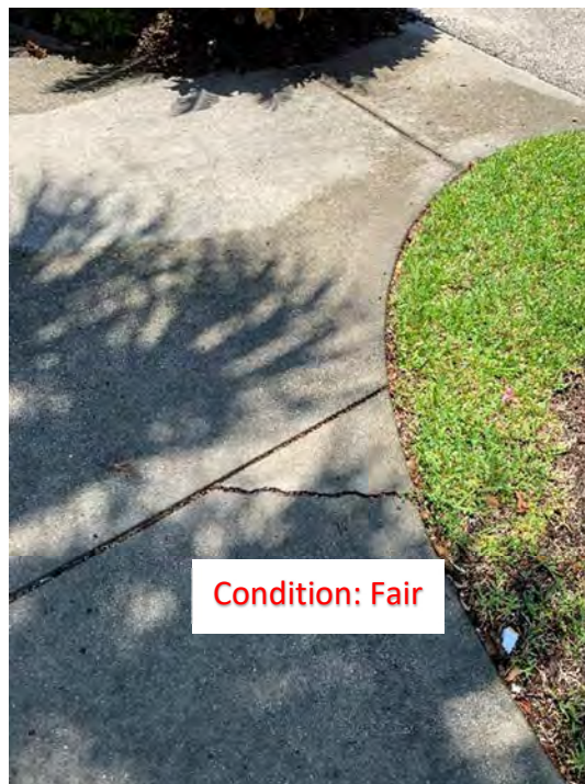
(294) Corner Crack
