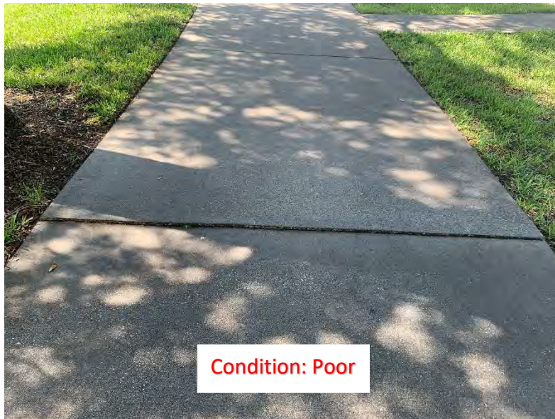
(233) Elevated Corner/Slab (1)
