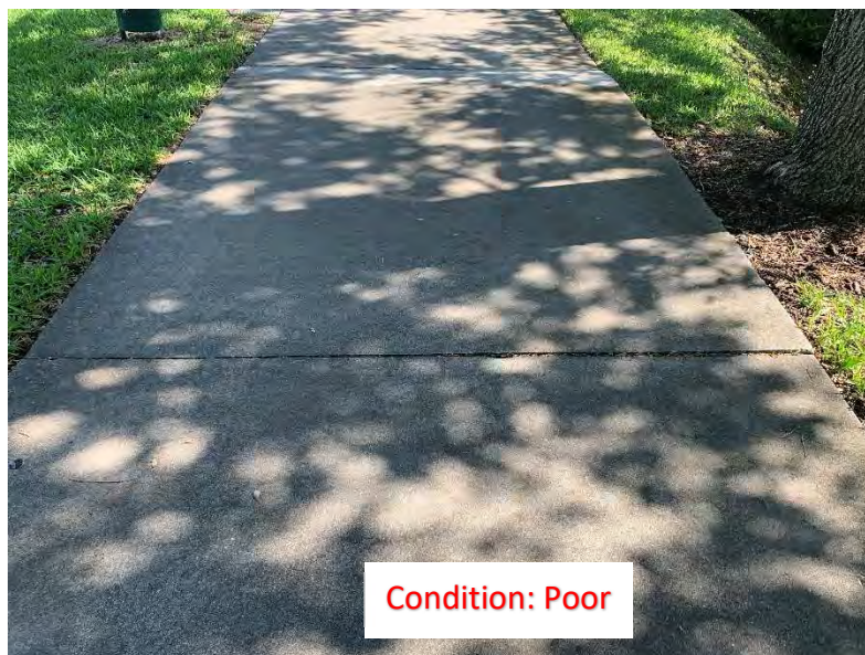
(239) Elevated Corner/Slab (2)
