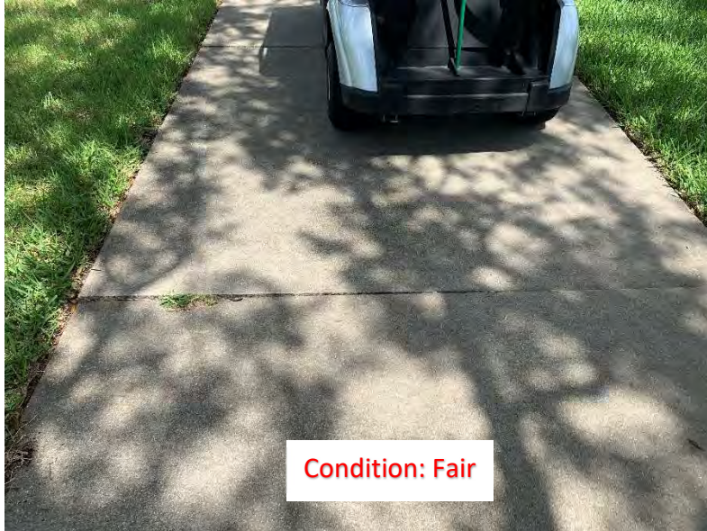
(269) Elevated Corner/Slab (1)
