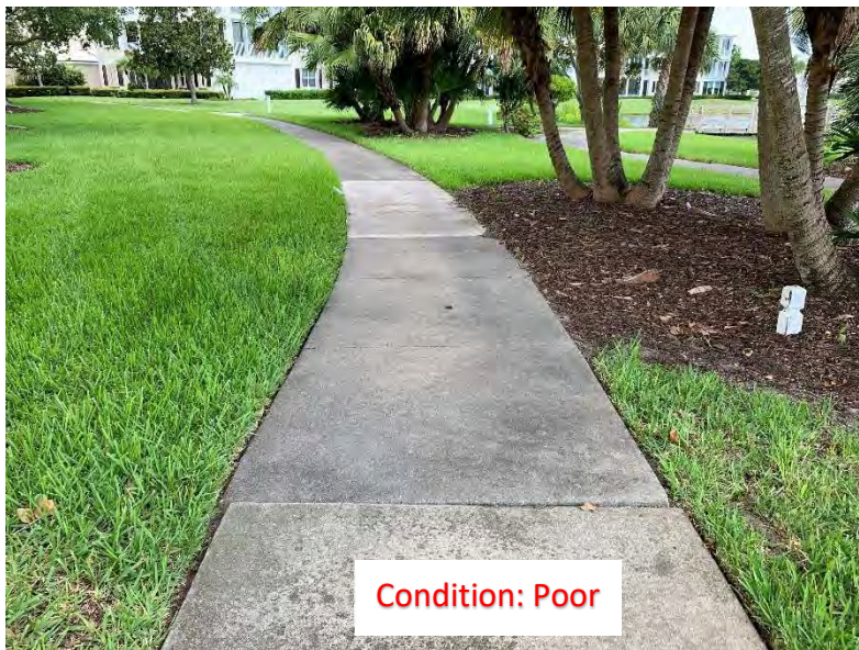
(271) Elevated Corner/Slab (1)
