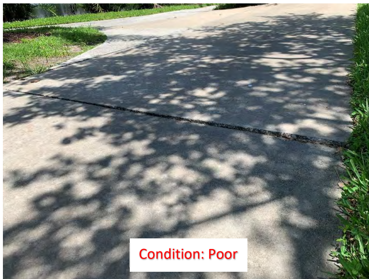
(302) Elevated Corner/Slab
