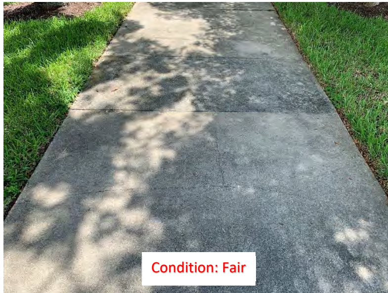
(256) Center and Corner Cracks
