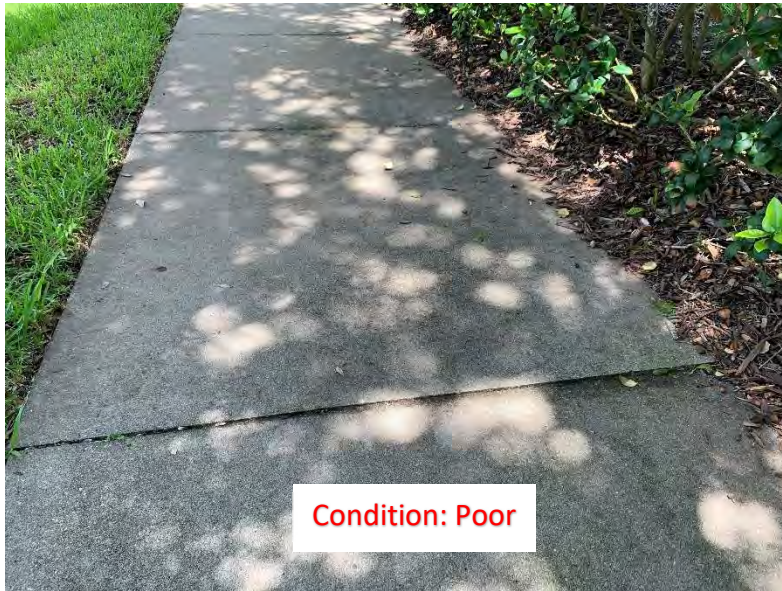
(274) Elevated Corner/Slab
