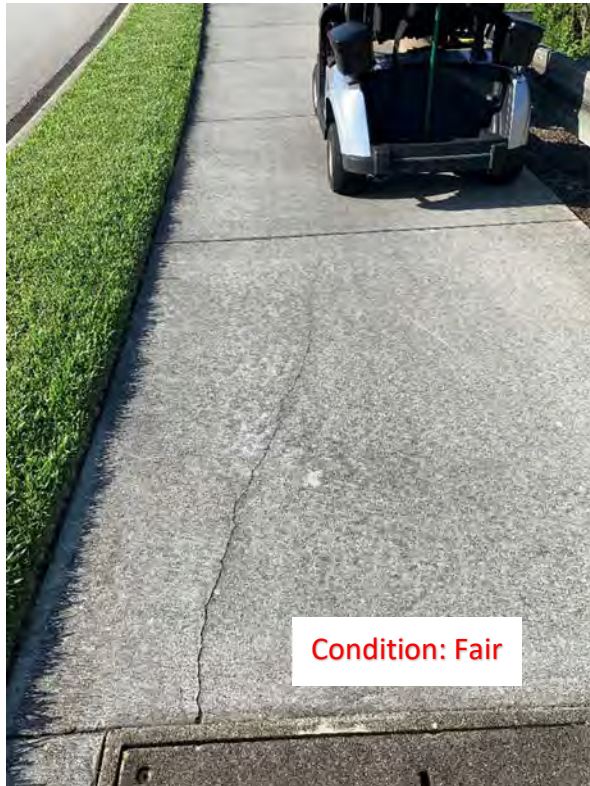
(174) Center Crack
