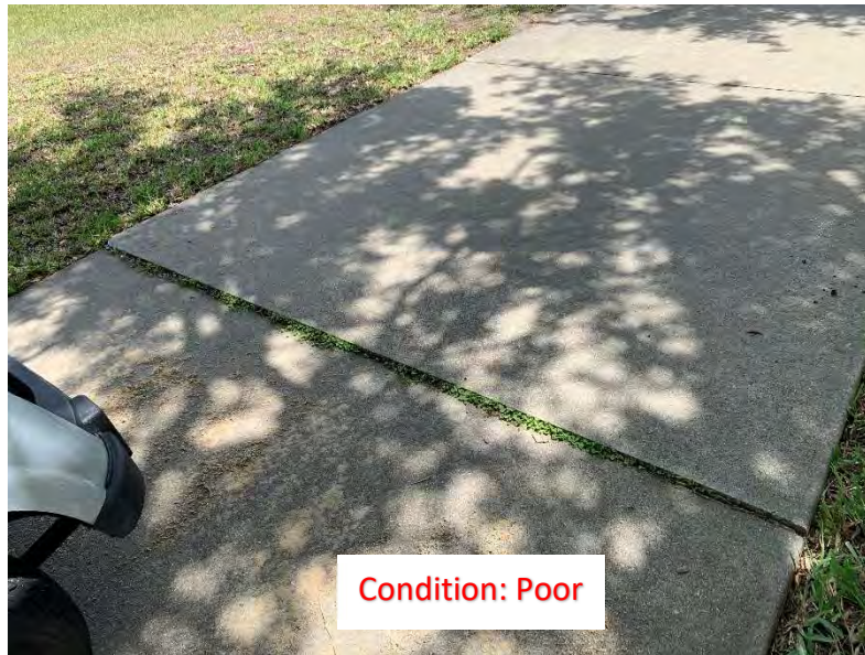
(266) Elevated Corner/Slab (2)
