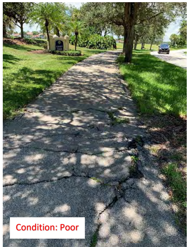
(1) Sidewalks Cracks (9)
