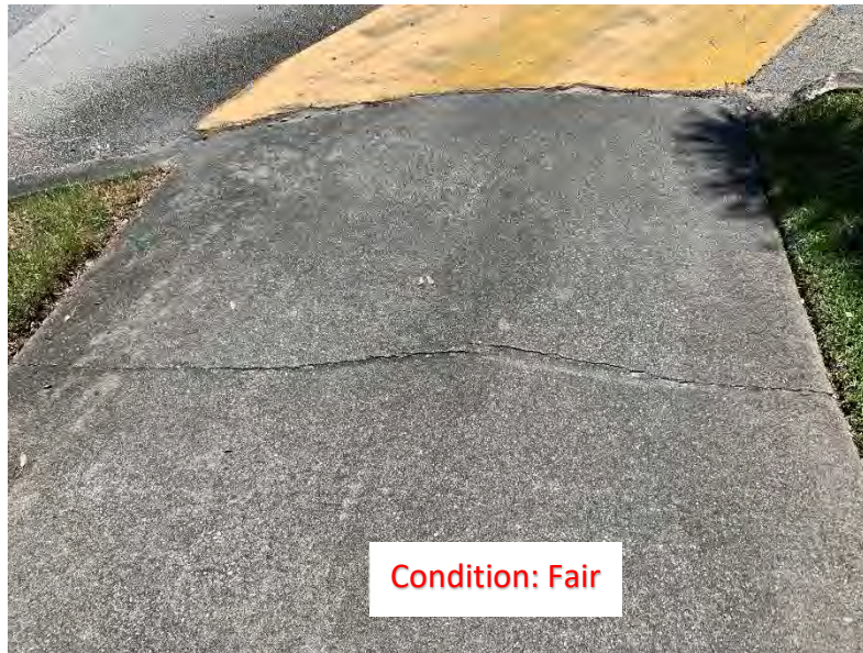
(284) Elevated Corners and Center Cracks (2)
