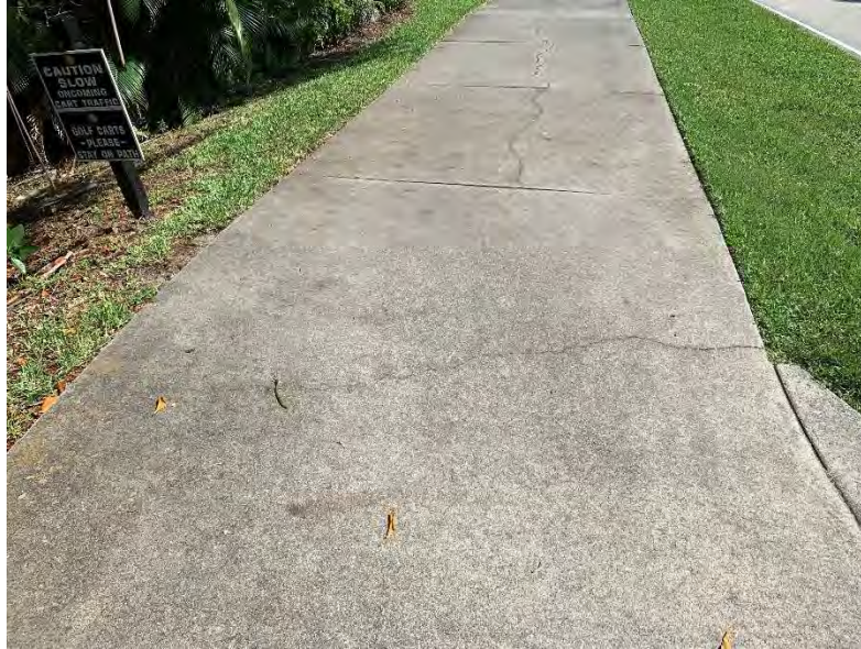
(241) Center Cracks (3)
