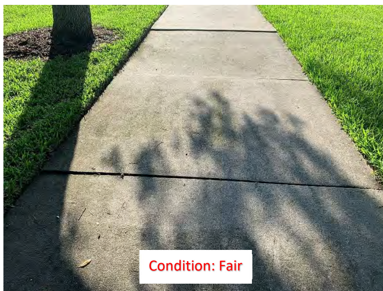
(157) Elevated Corner/Slab
