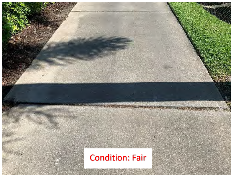
(245) Elevated Corner/Slab
