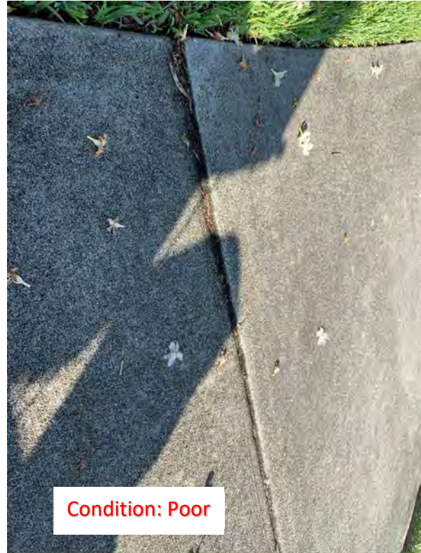
(171) Elevated Corner/Slab
