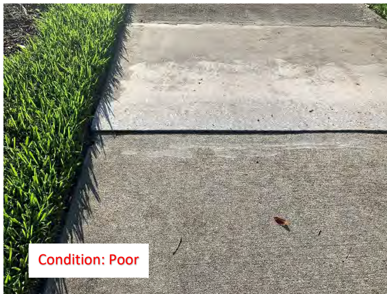
(151) Elevated Corner/Slab
