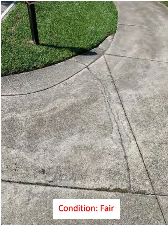
(241) Center Cracks (1)
