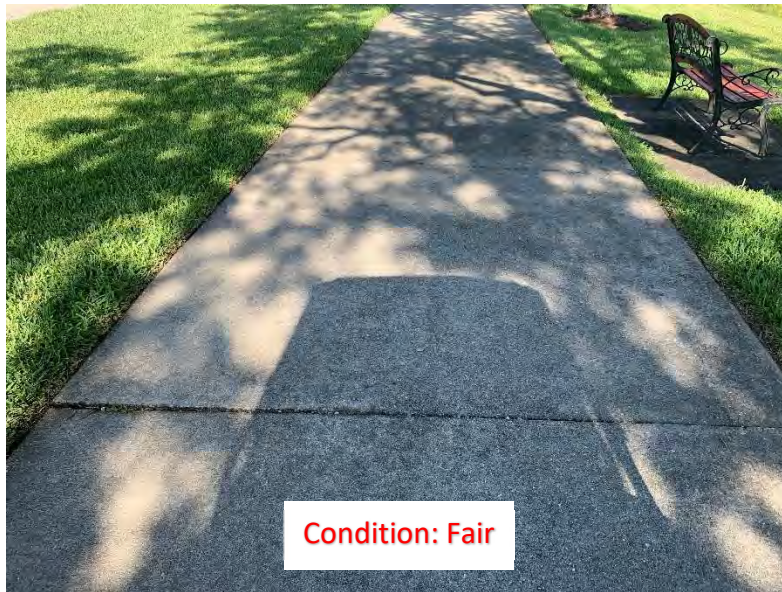
(203) Elevated Corner/Slab
