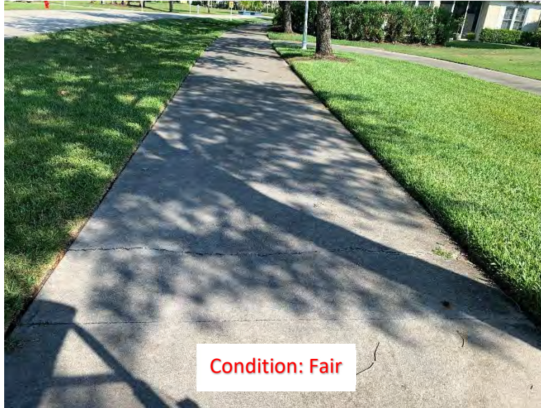
(208) Center Crack
