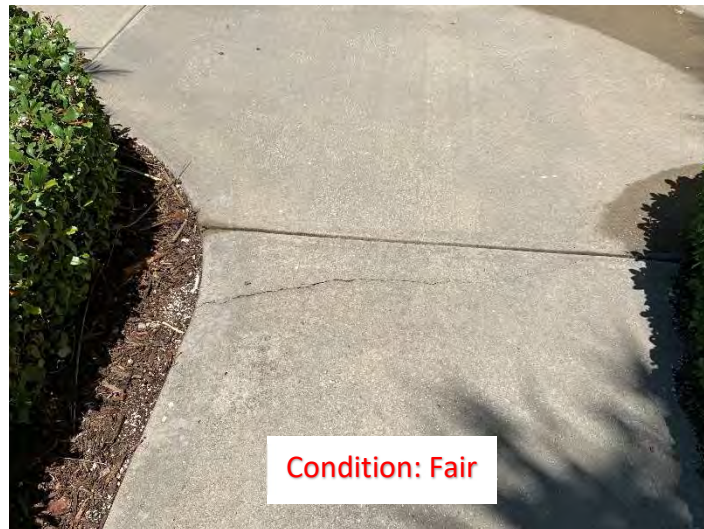
(296) Corner Crack
