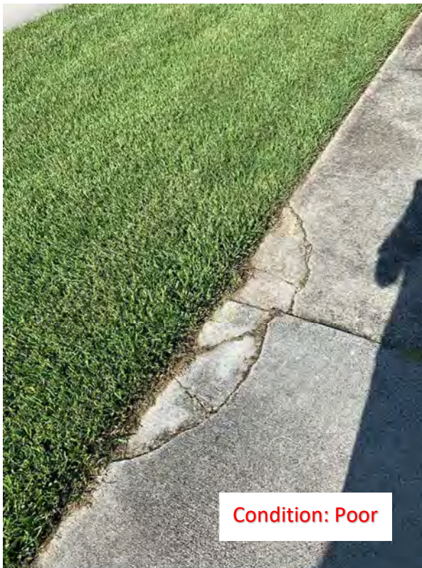
(191) Corner Cracks (1)
