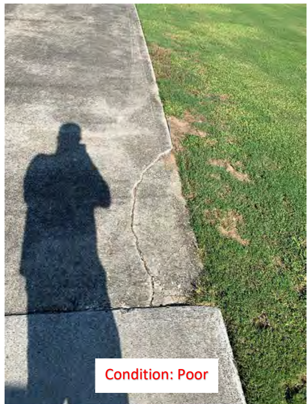
(191) Corner Cracks (2)
