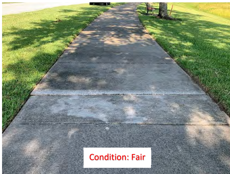
(202) Elevated Corner/Slab (1)
