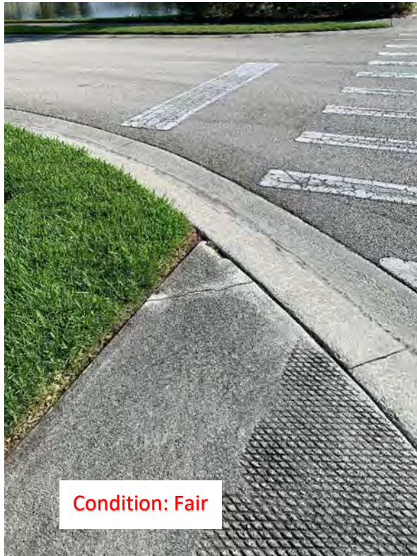
(185) Corner Crack
