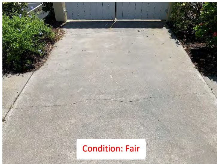
(297) Center Cracks (1)
