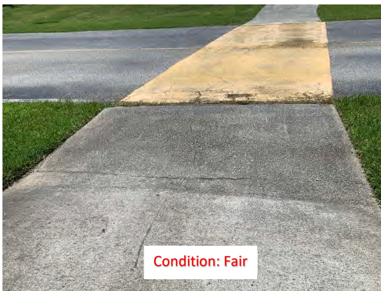
(284) Elevated Corners and Center Cracks (1)
