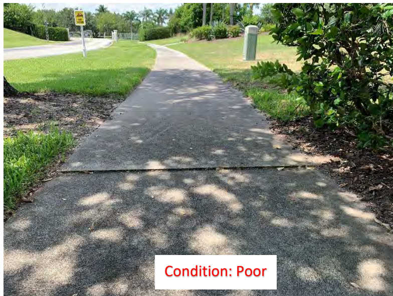
(282) Elevated Corner/Slab
