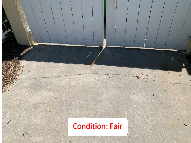
(297) Center Cracks (2)
