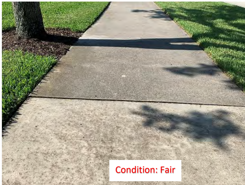
(216) Elevated Corner/Slab (2)
