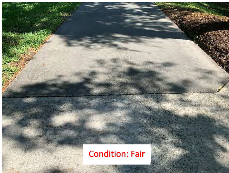
(233) Elevated Corner/Slab (2)
