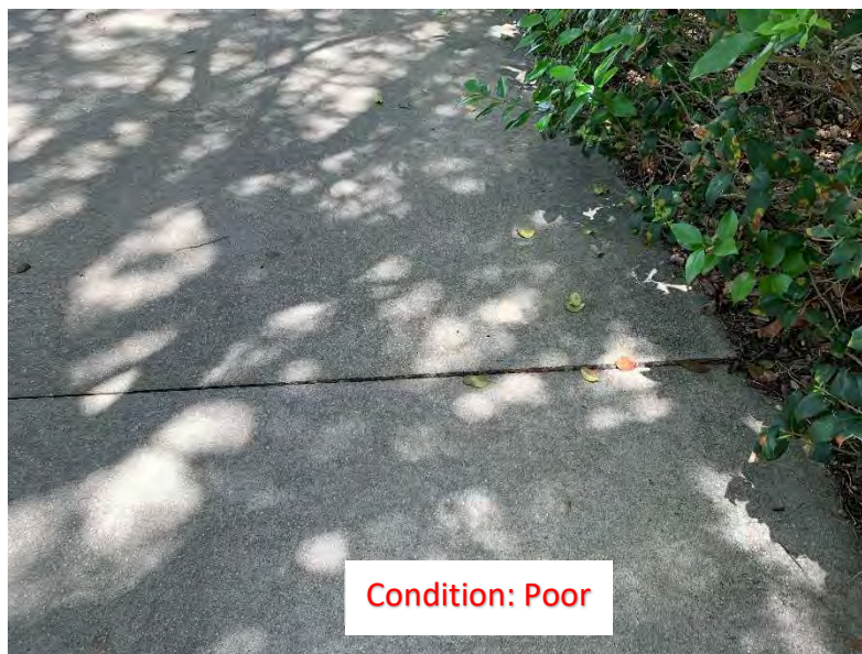
(266) Elevated Corner/Slab (3)
