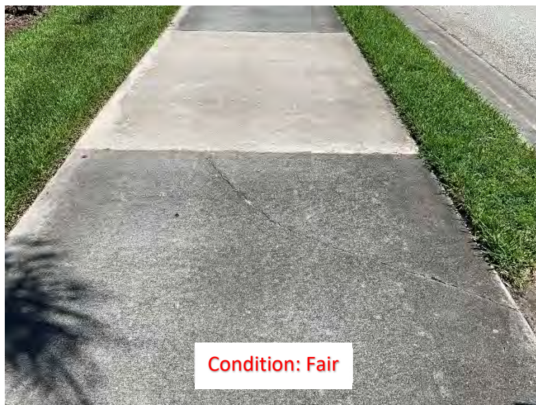
(288) Corner Cracks
