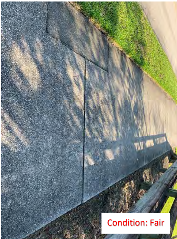
(168) Elevated Corner/Slab
