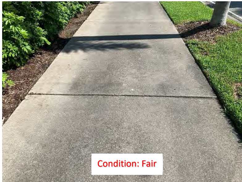
(244) Elevated Corner/Slab
