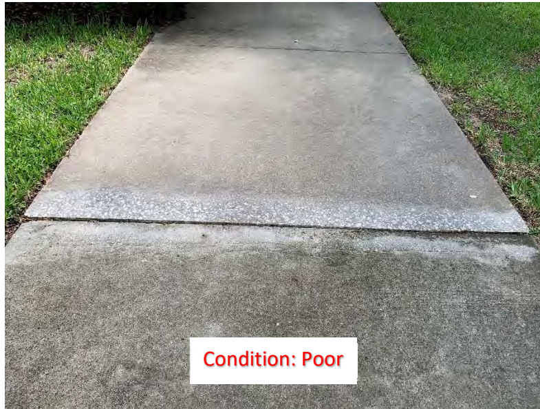
(267) Elevated Corner/Slab (1)
