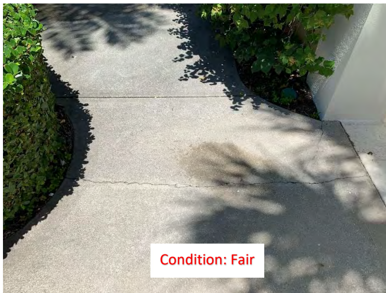
(292) Center Cracks (2)
