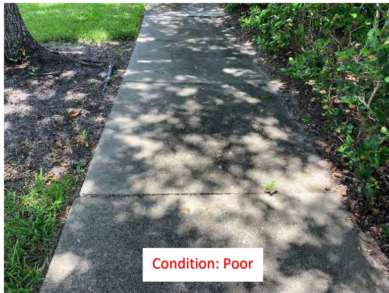
(280) Elevated Corner/Slab
