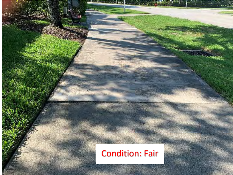
(212) Elevated Corner/Slab
