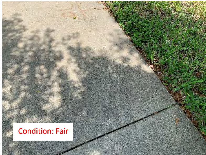
(258) Corner Cracks (1)
