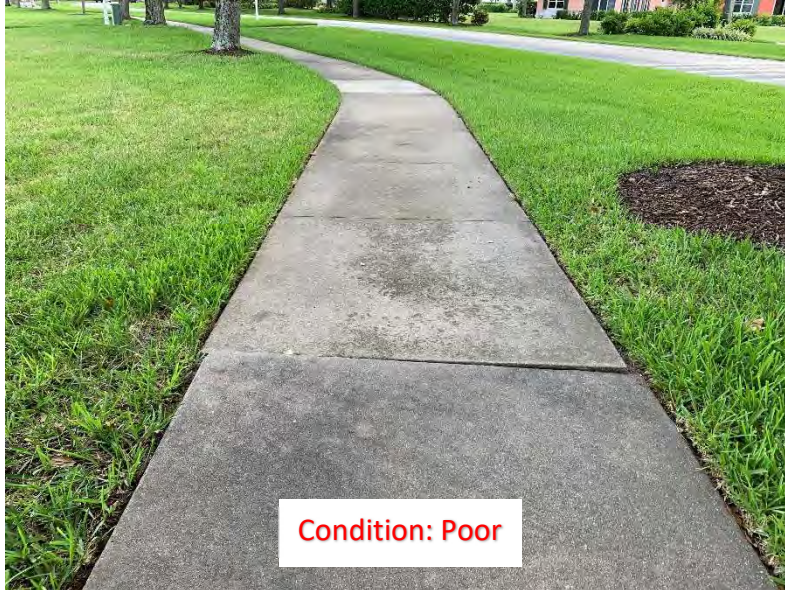
(271) Elevated Corner/Slab (2)
