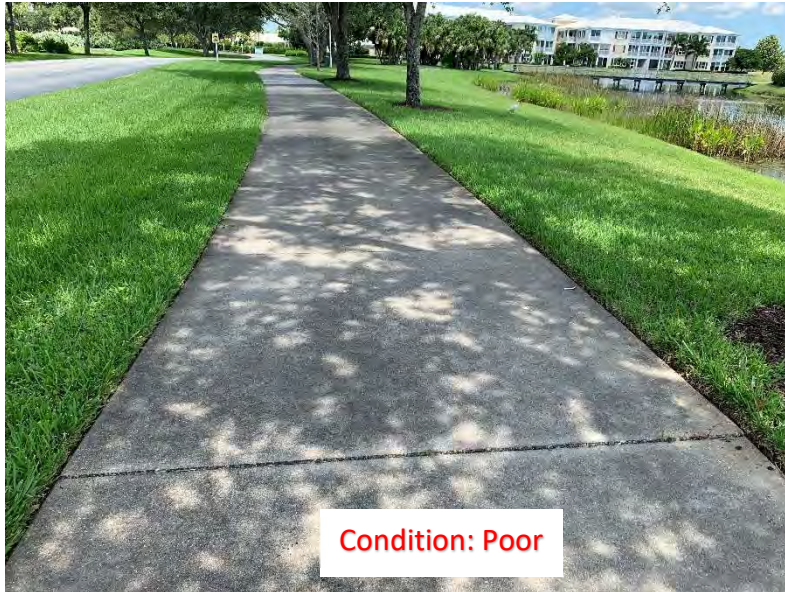
(270) Elevated Corner/Slab (2)
