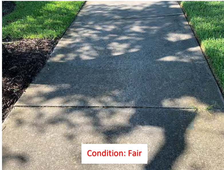
(214) Elevated Corner/Slab
