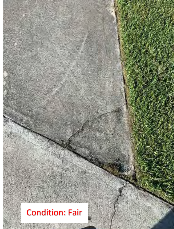
(179) Corner Crack
