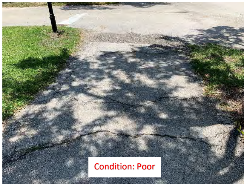
(1) Sidewalk Cracks (5)
