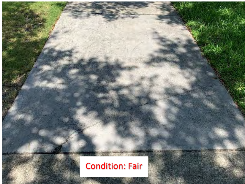
(301) Corner Crack
