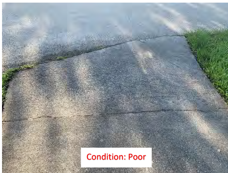
(152) Center Cracks and Corner Crack (2)
