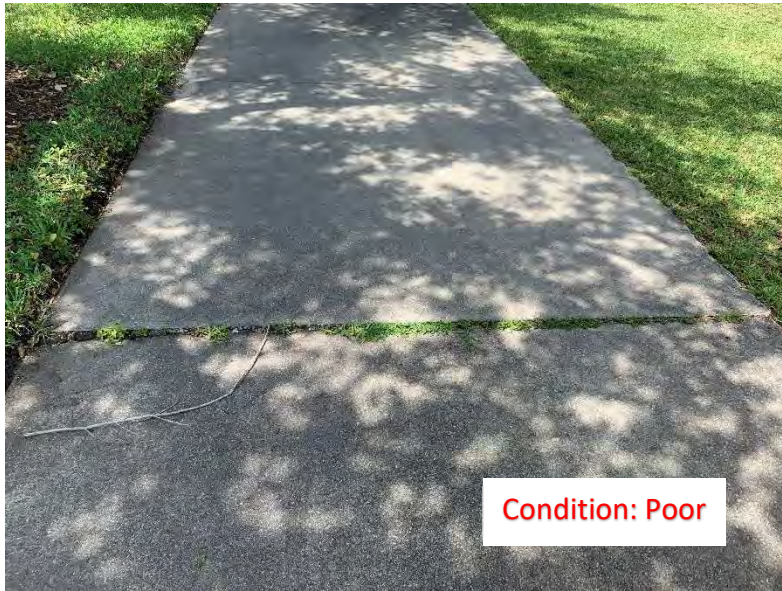
(266) Elevated Corner/Slab (1)
