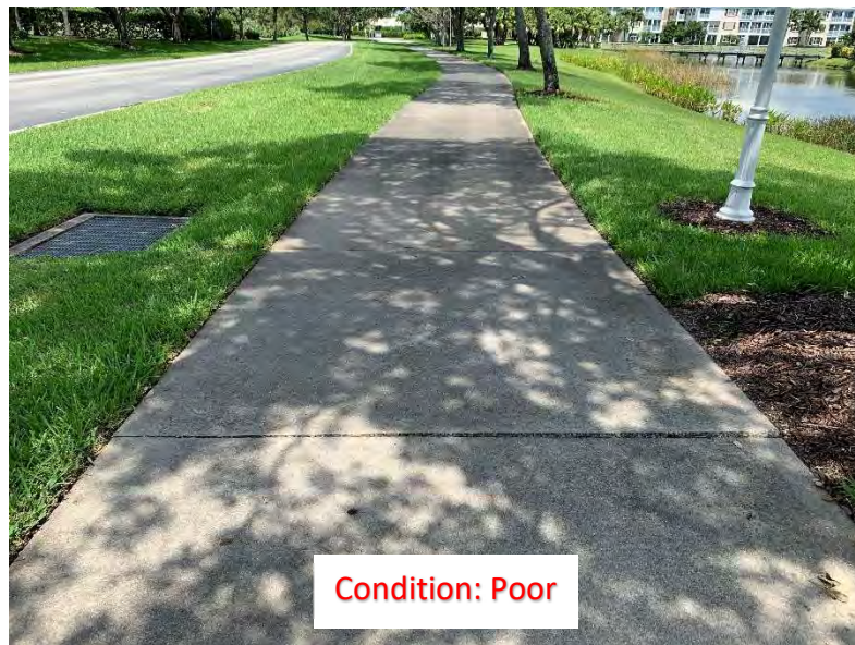
(270) Elevated Corner/Slab (1)
