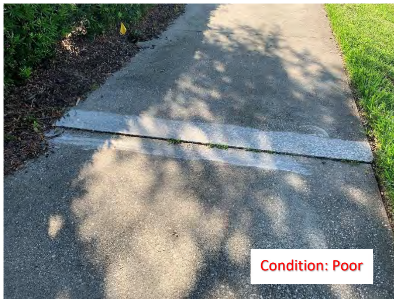
(195) Elevated Corner/Slab (2)
