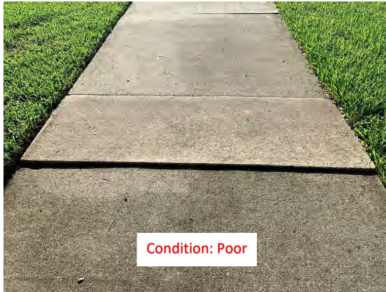
(158) Elevated Corner/Slab
