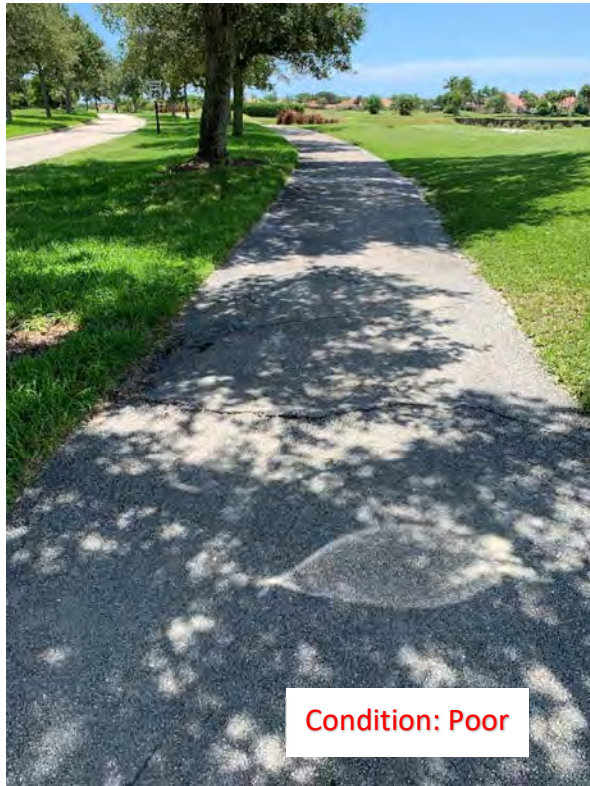
(1) Sidewalks Cracks (6)
