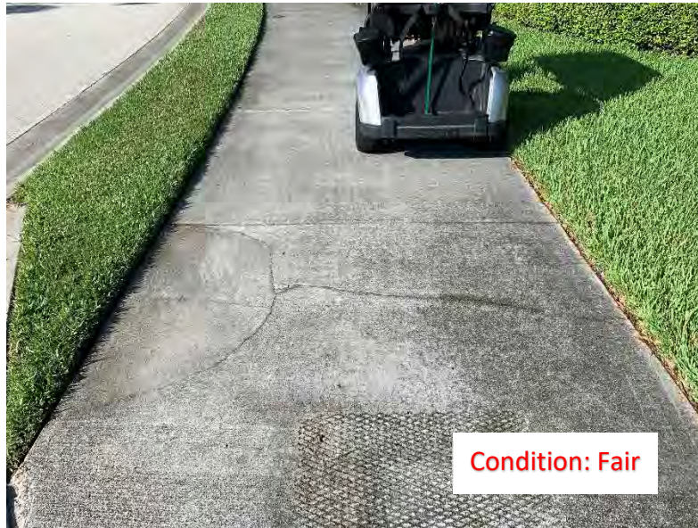
(187) Center Cracks (2)
