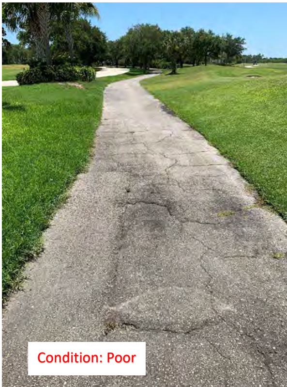
(1) Sidewalks Cracks (8)
