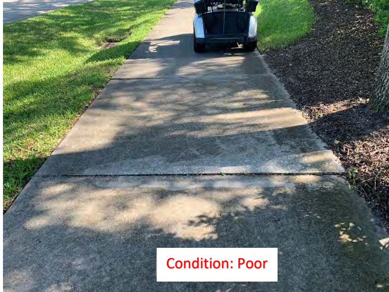
(218) Elevated Corner/Slab (1)
