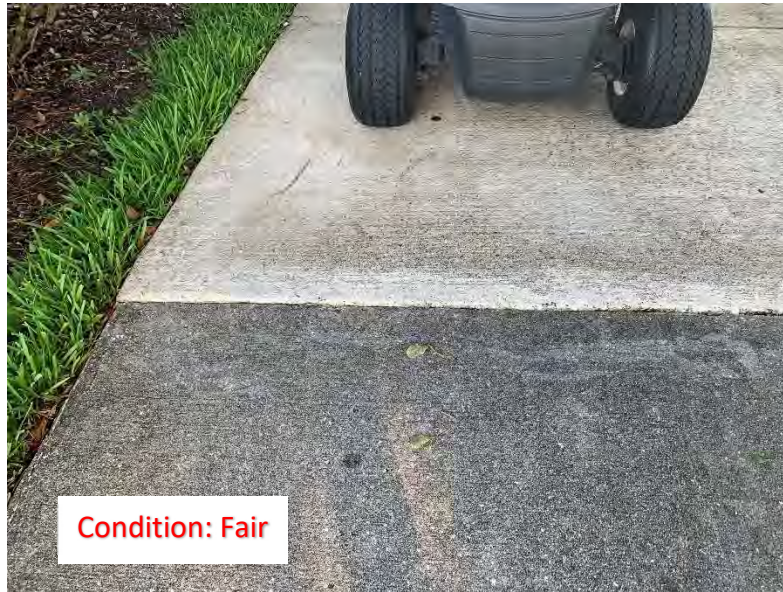
(149) Elevated Corner/Slab (1)
