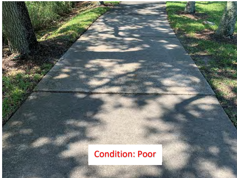
(239) Elevated Corner/Slab (1)
