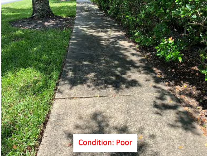
(279) Elevated Corner/Slab
