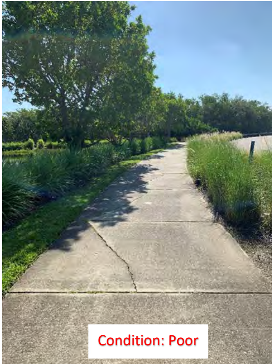
(228) Center Cracks (2)
