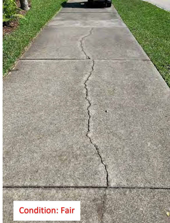
(241) Center Cracks (5)
