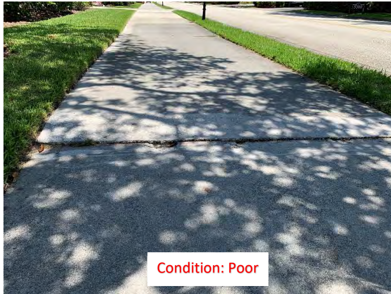
(289) Elevated Corner/Slab
