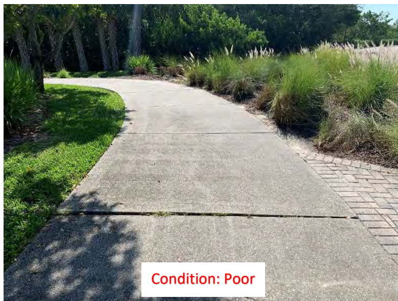
(230) Elevated Corner/Slab
