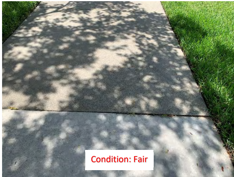
(268) Elevated Corner/Slab (2)
