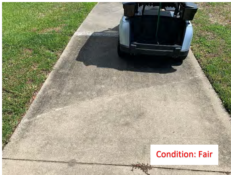
(252) Center Crack
