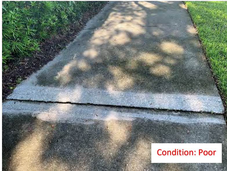
(194) Elevated Corner/Slab (1)
