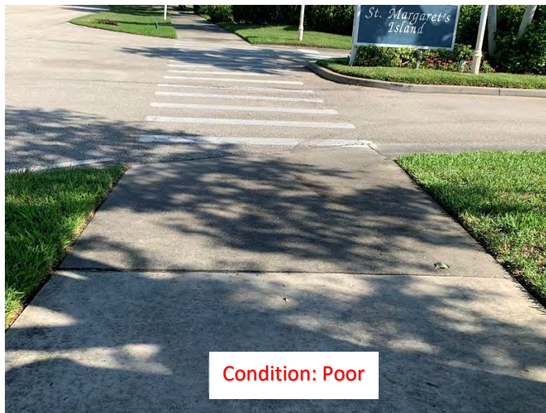
(222) Elevated Corner/Slab (2)
