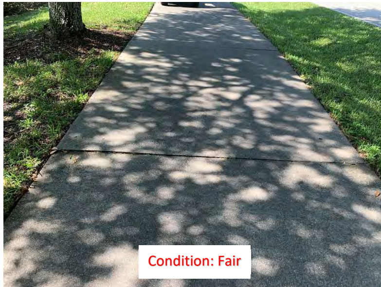
(237) Elevated Corner/Slab
