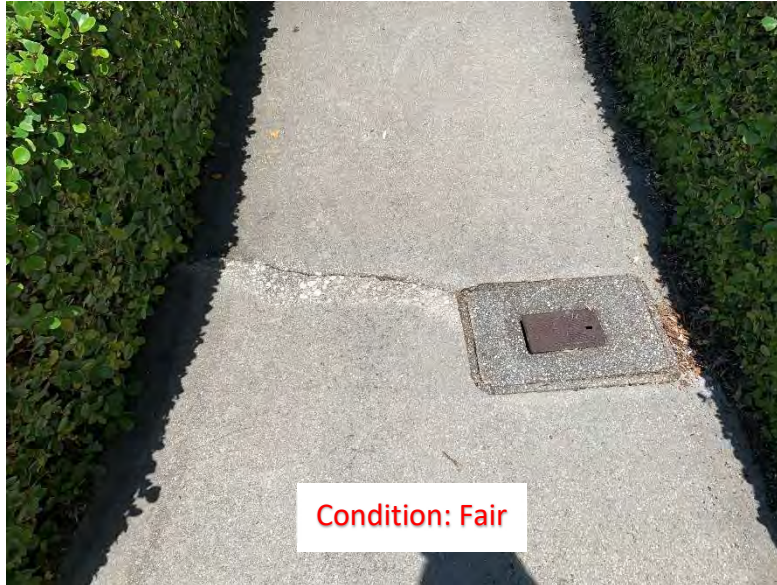
(292) Center Cracks (1)
