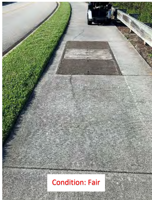
(173) Center Crack
