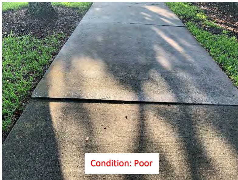
(156) Elevated Corner/Slab (1)
