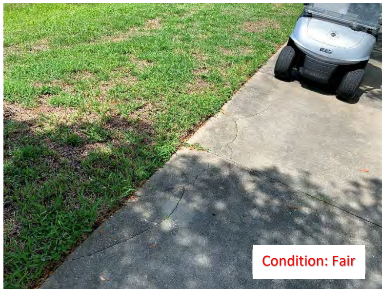
(255) Corner Cracks (2)
