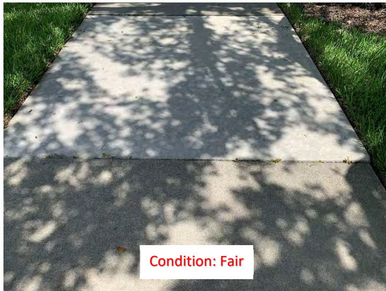
(268) Elevated Corner/Slab (1)
