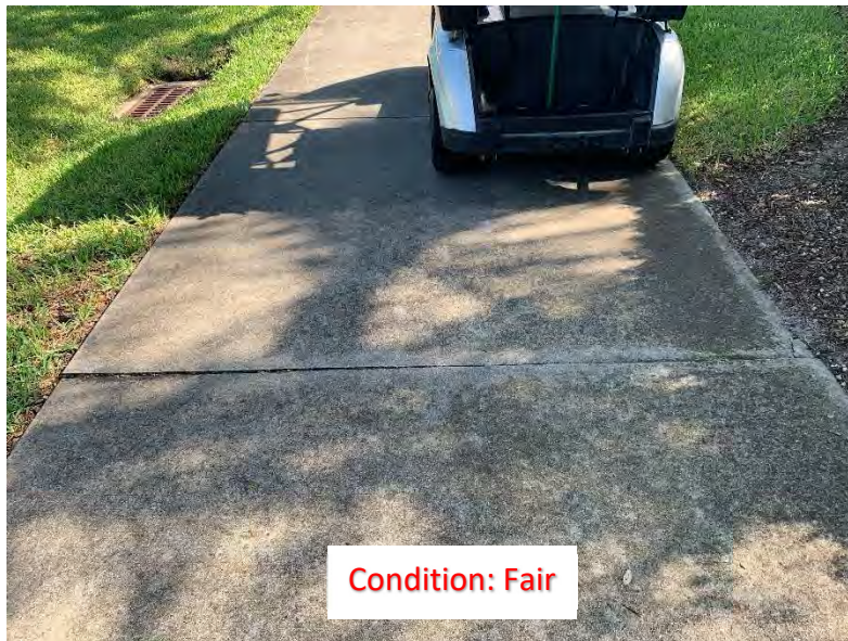
(218) Elevated Corner/Slab (2)
