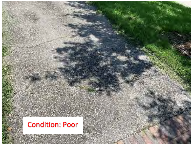
(1) Sidewalk Cracks (1)
