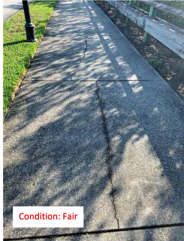
(167) Center Crack
