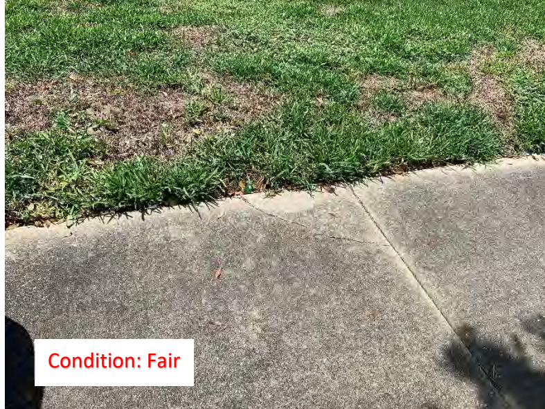
(255) Corner Cracks (1)
