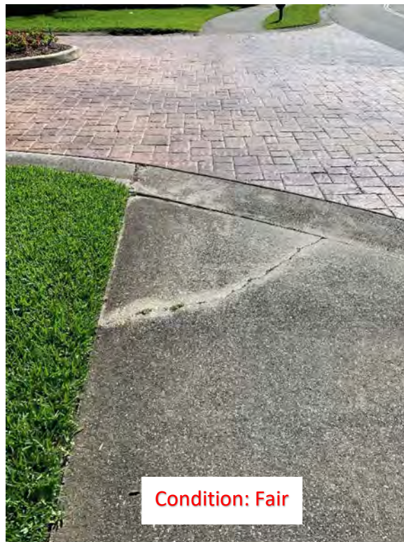
(227) Corner Crack
