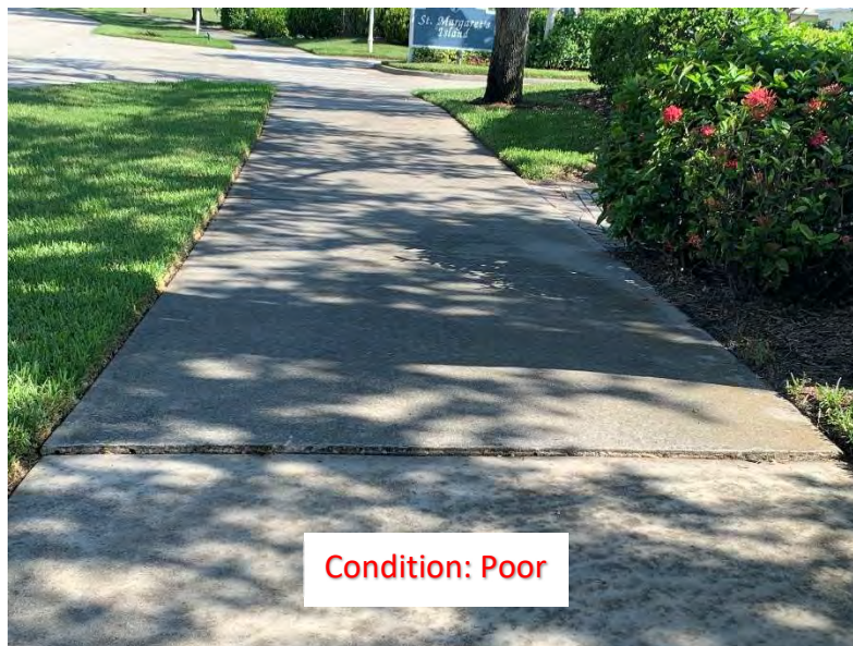
(221) Elevated Corner/Slab (2)
