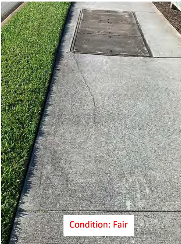
(176) Center Crack
