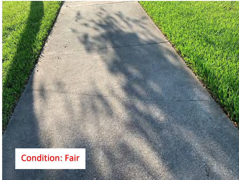
(150) Center Crack
