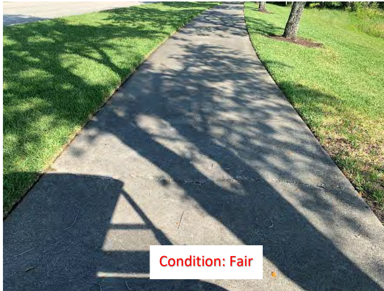
(204) Center Crack
