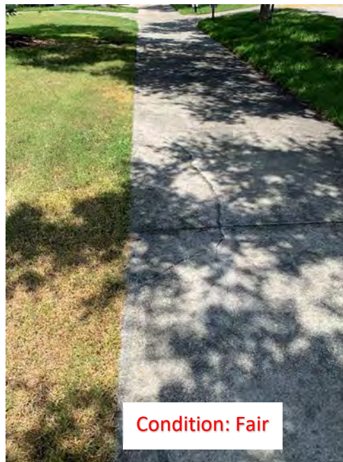
(299) Corner Cracks
