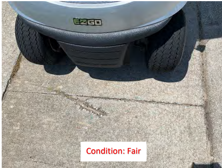
(283) Center Crack and Chipped Concrete
