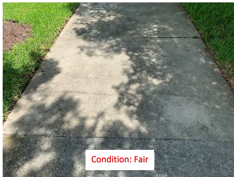
(257) Center and Corner Cracks
