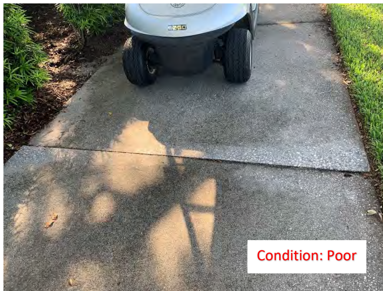
(194) Elevated Corner/Slab (2)
