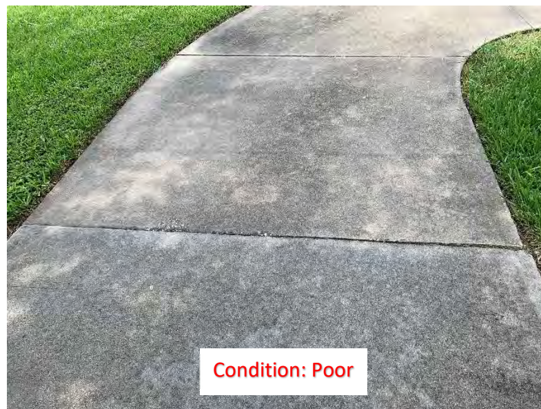
(267) Elevated Corner/Slab (2)
