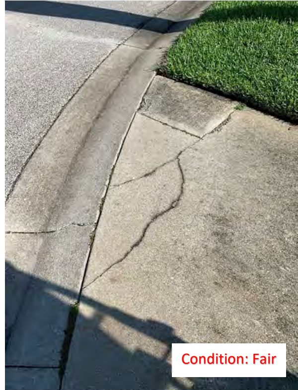
(197) Center Cracks
