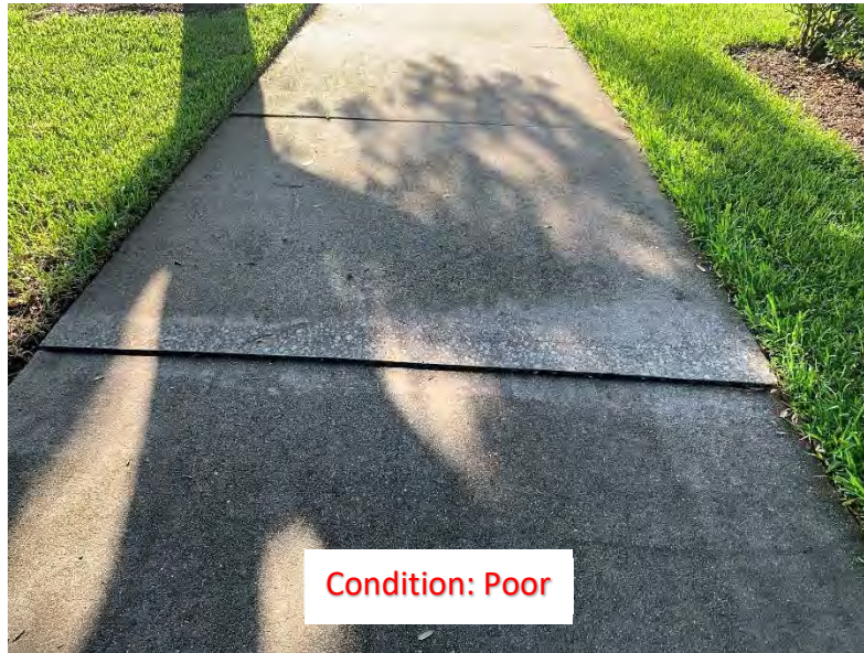
(156) Elevated Corner/Slab (2)
