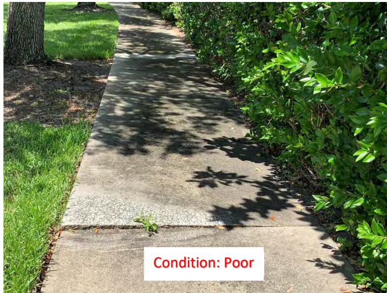
(277) Elevated Corner/Slab
