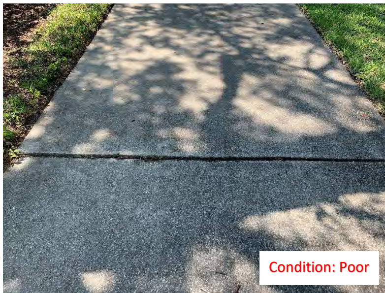
(107) Elevated Corner/Slab
