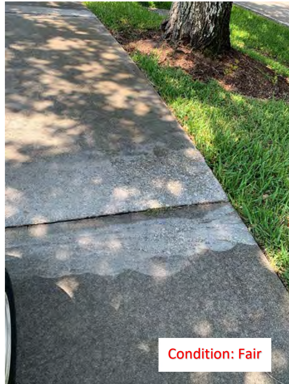
(147) Elevated Corner/Slab
