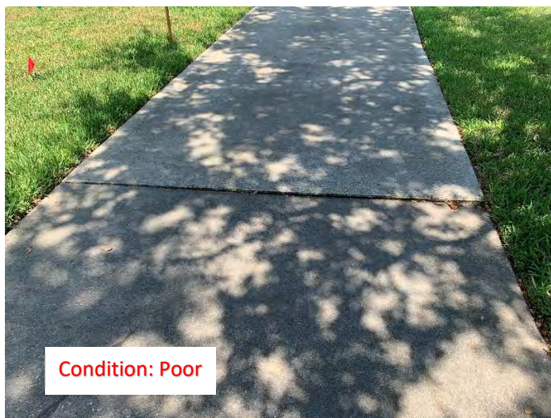
(142) Elevated Corner/Slab
