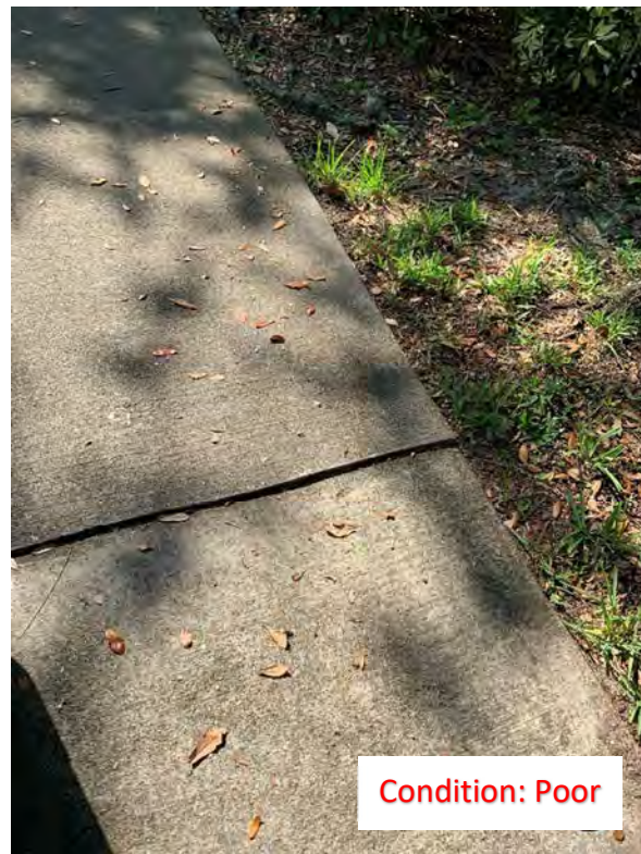
(69) Elevated Corner/Slab
