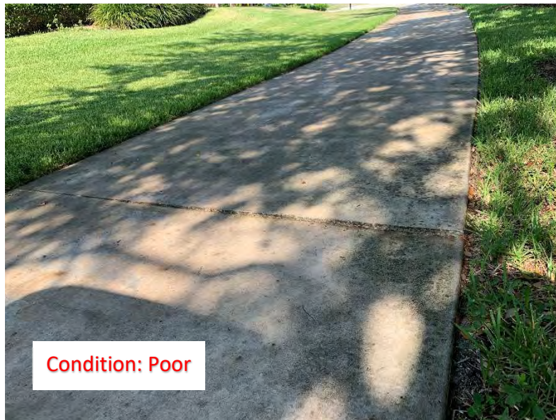
(71) Elevated Corner/Slab
