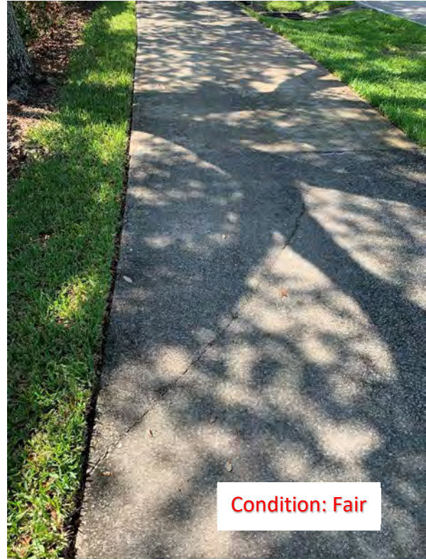
(90) Corner Crack
