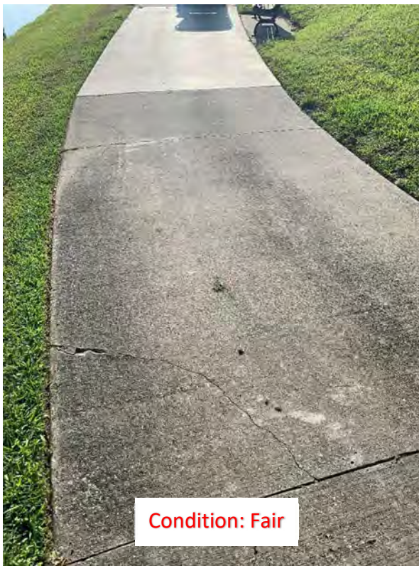
(3) Corner and Center Crack
