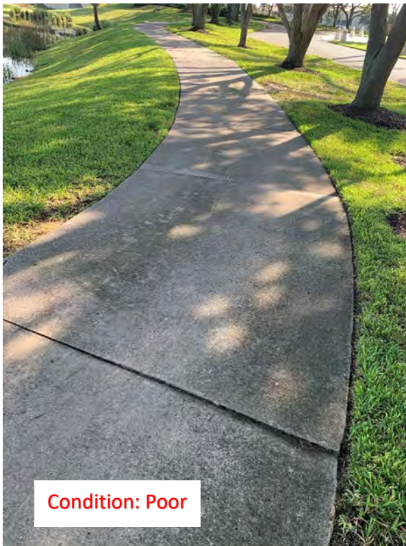
(22) Elevated Corner/Slab
