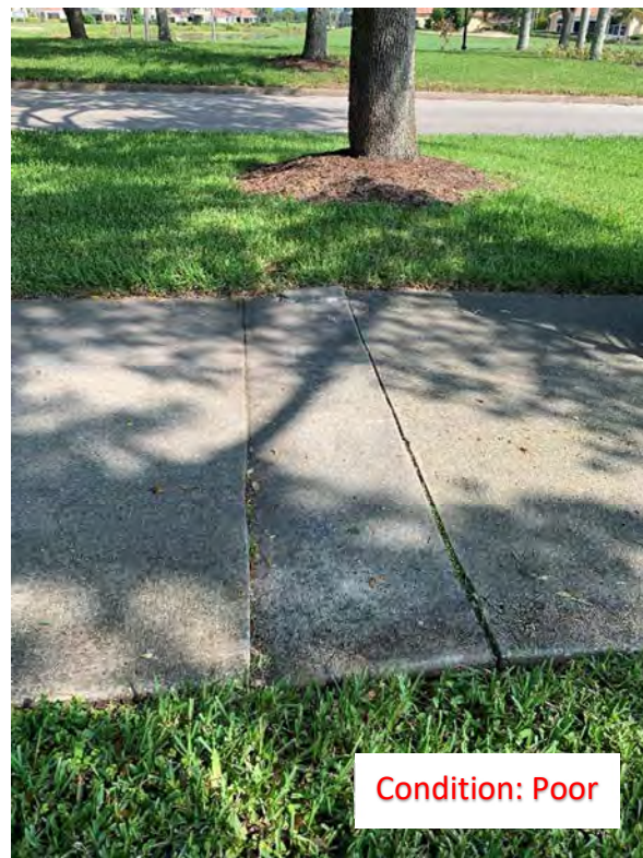
(73) Elevated Corner/Slab (1)
