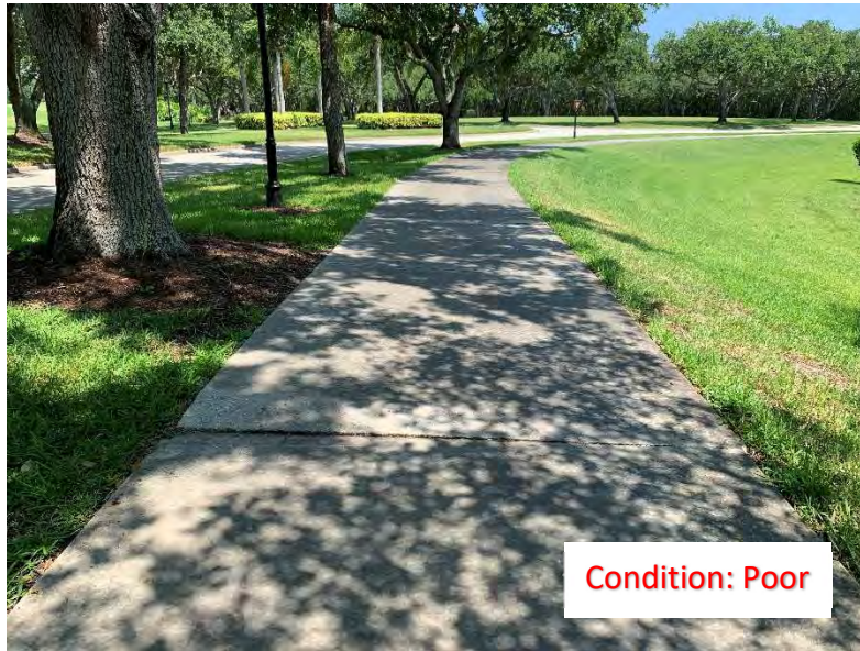
(145) Elevated Corner/Slab
