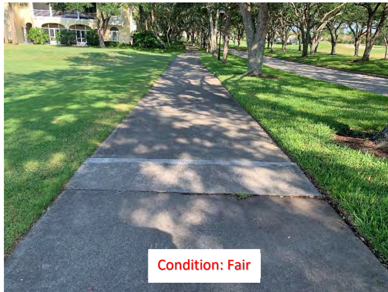
(65) Elevated Corner/Slab
