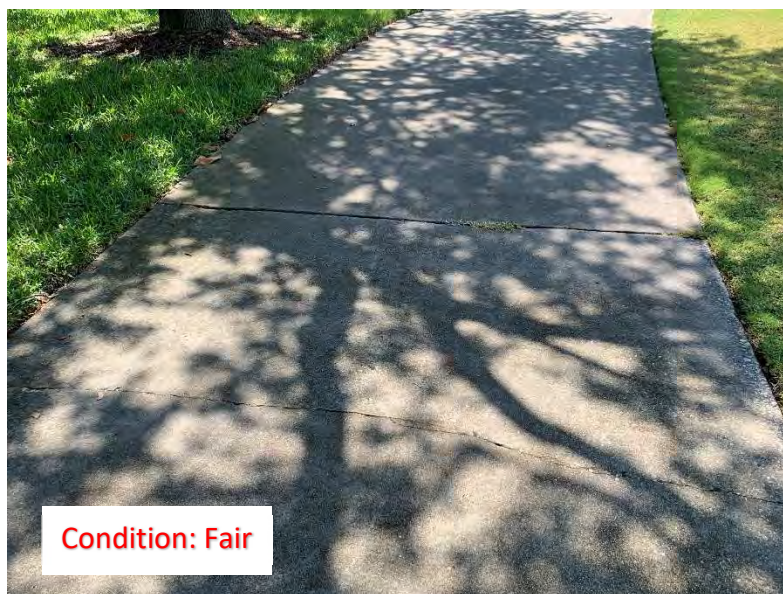
(128) Center Cracks (1)
