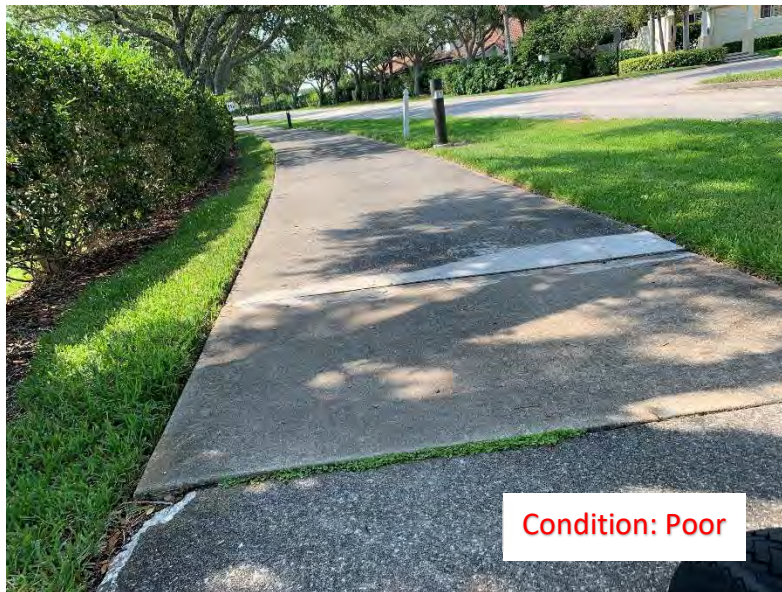
(96) Elevated Corner/Slab
