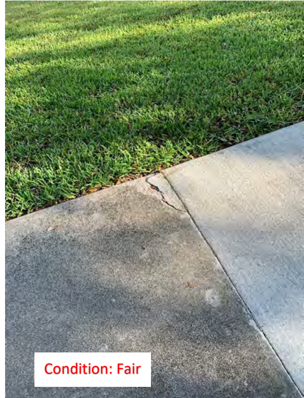
(31) Corner Crack
