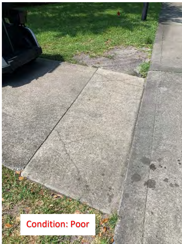
(140) Elevated Corners, Corner and Center Cracks (6 and 7)
