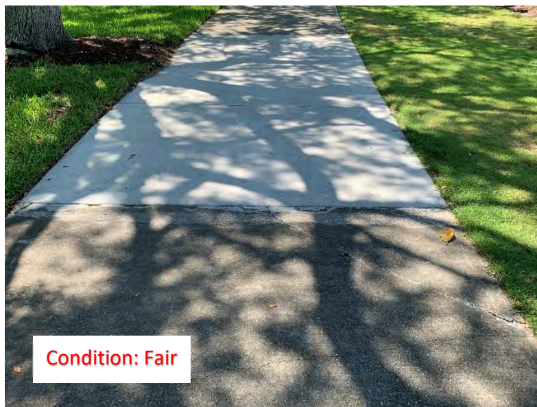
(129) Corner Cracks
