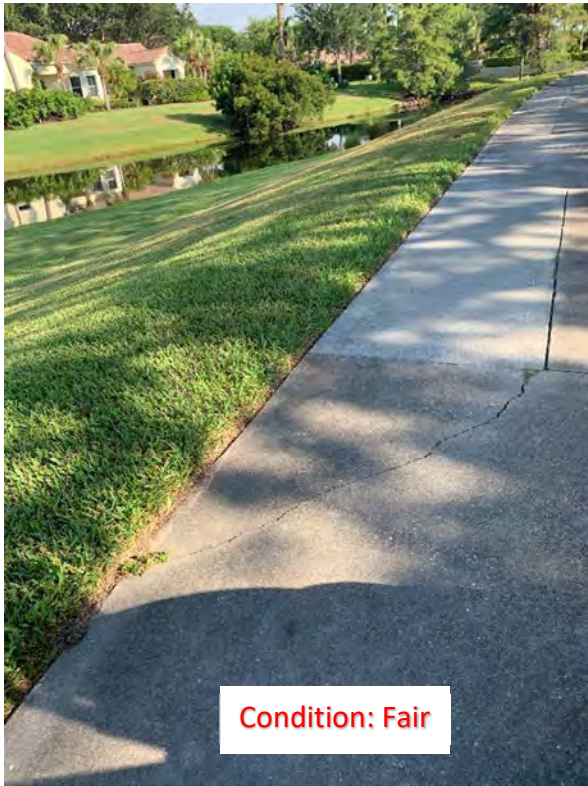
(35) Corner Crack
