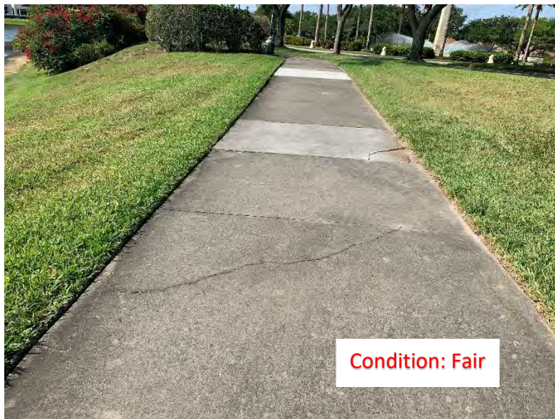
(87) Corner Cracks (1)
