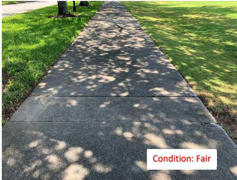
(133) Elevated Corner/Slab
