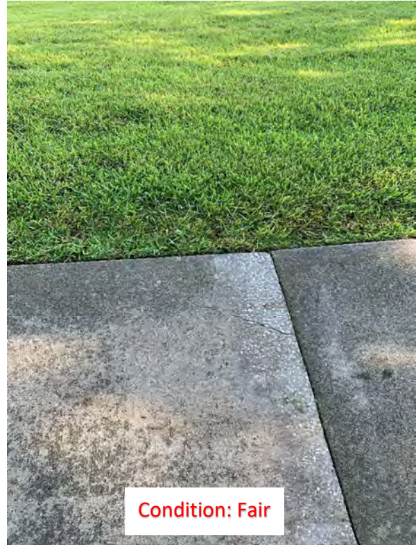
(21) Corner Crack
