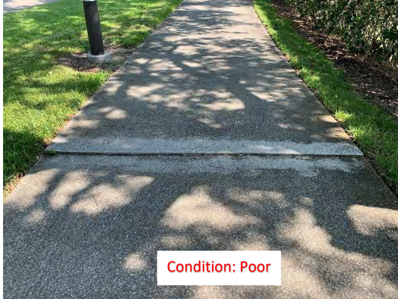
(95) Elevated Corner/Slab
