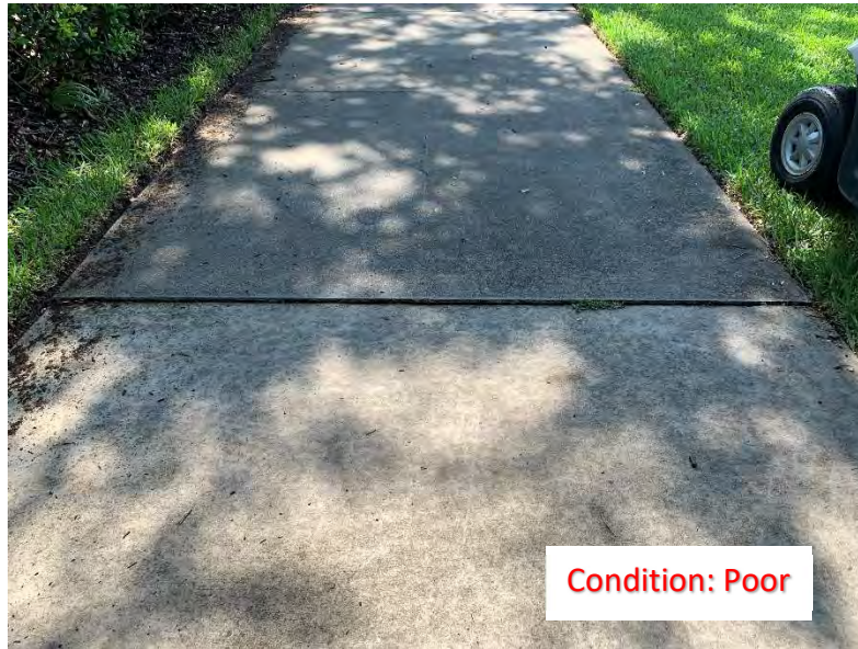
(110) Elevated Corner/Slab
