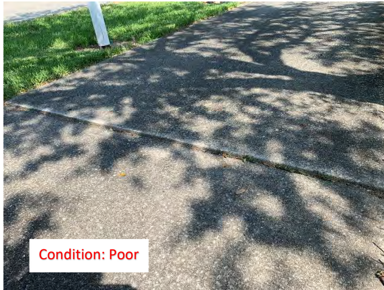
(97) Elevated Corner/Slab
