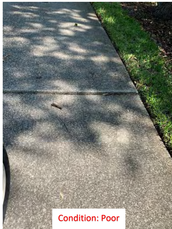
(94) Elevated Corner/Slab
