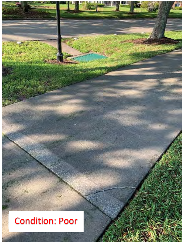
(24) Corner Crack
