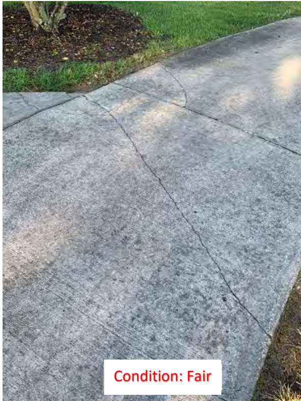
(1) Corner and Center Crack
