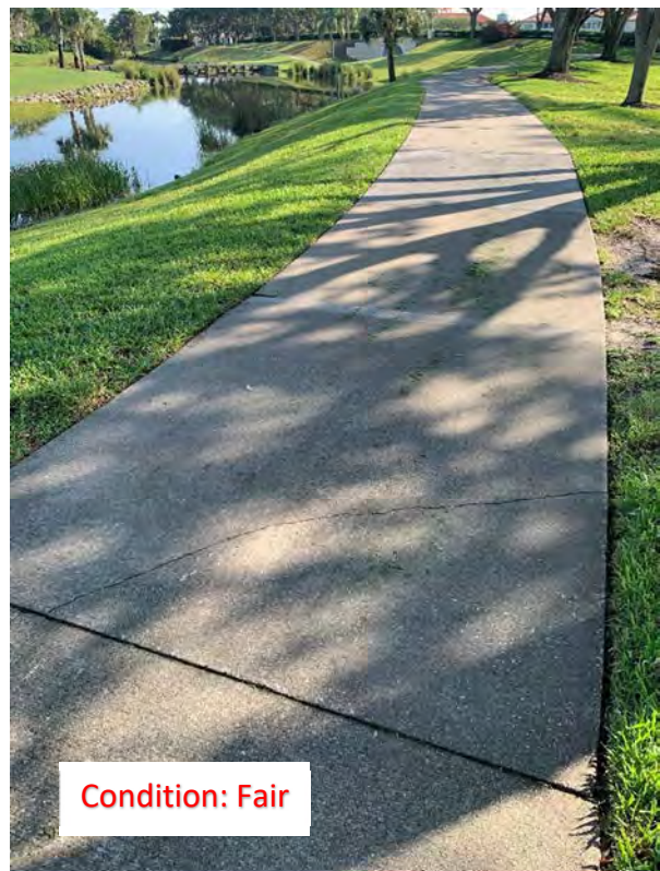
(23) Corner Crack
