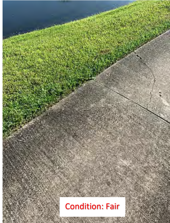
(2) Corner Crack
