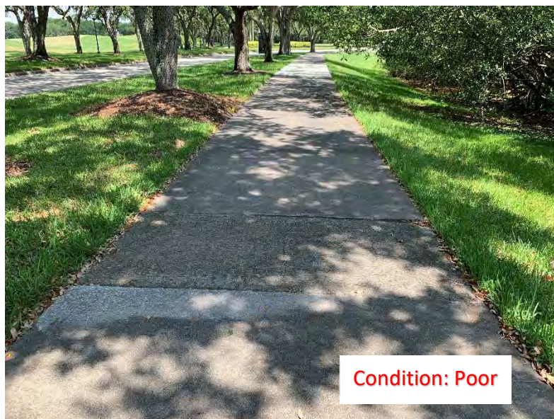
(144) Elevated Corner/Slab
