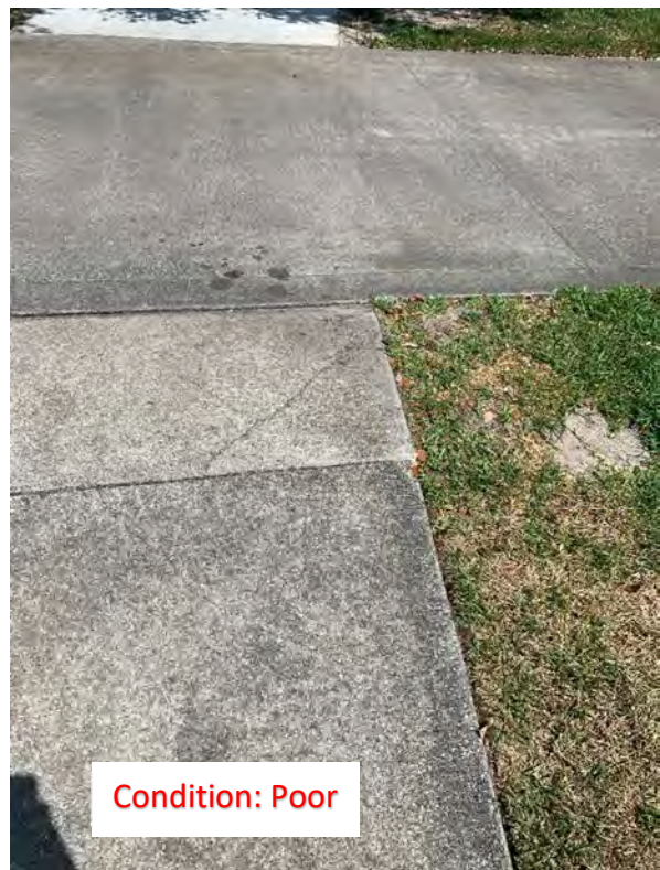
(140) Elevated Corners, Corner and Center Cracks (6 and 7)
