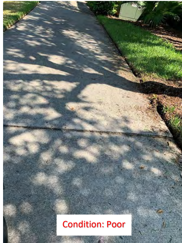
(119) Elevated Corner/Slab
