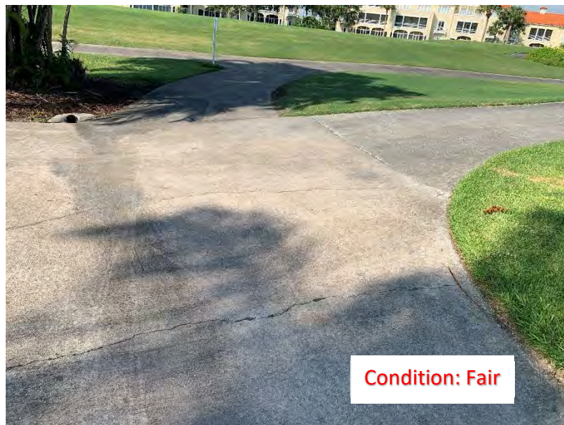
(61) Center Cracks (2)
