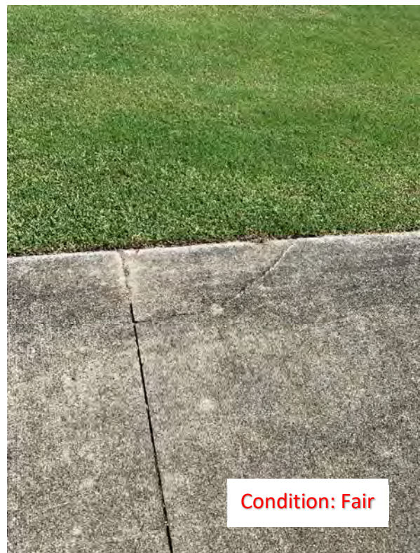
(114) Corner Cracks (1)
