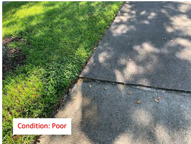
(68) Elevated Corner/Slab
