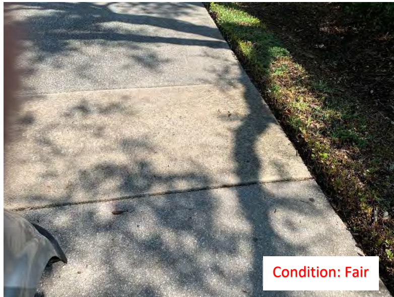
(108) Elevated Corner/Slab
