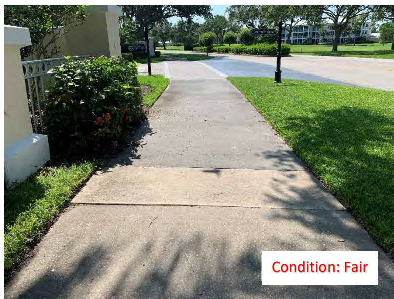
(109) Elevated Corner/Slab
