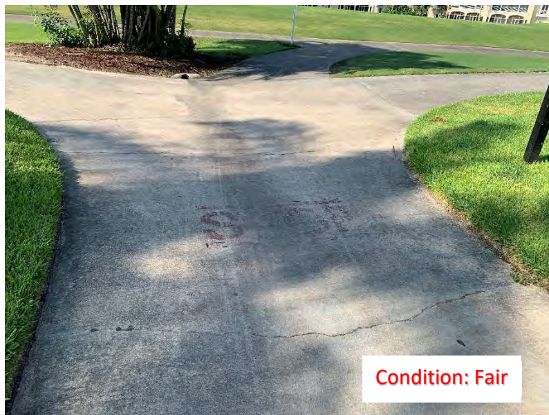
(60) Center Cracks (2)
