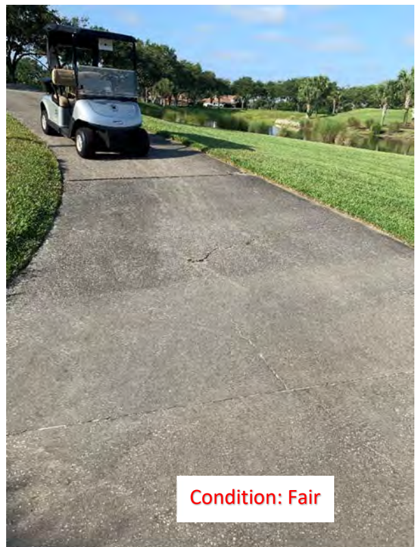
(34) Center Cracks (3)
