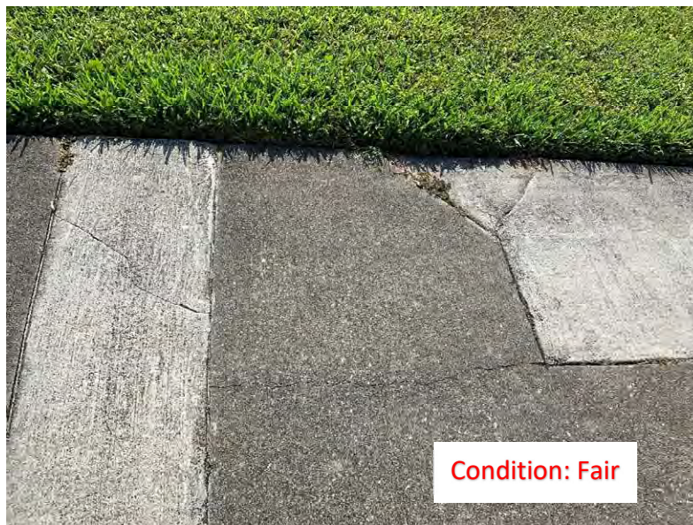
(85) Center Cracks
