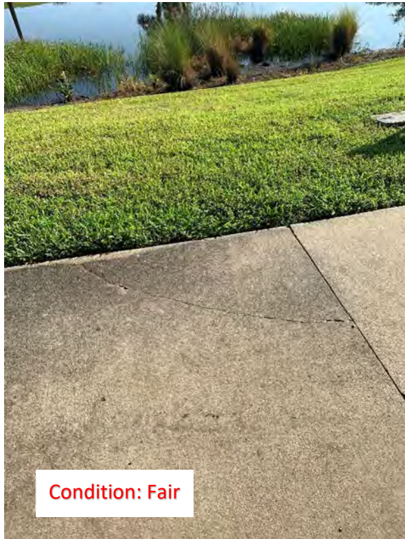
(16) Corner Crack
