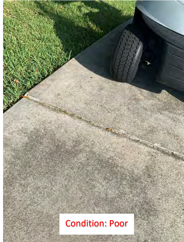
(6) Elevated Corner/Slab
