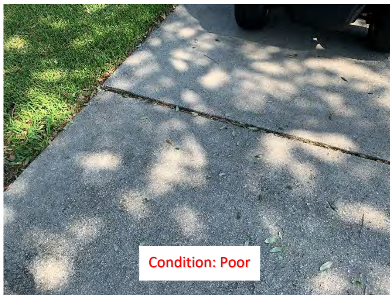
(91) Elevated Corner/Slab
