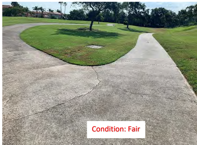
(58) Center Cracks
