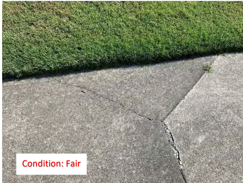
(62) Corner Cracks
