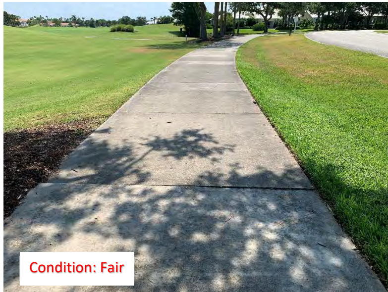
(112) Elevated Corner/Slab
