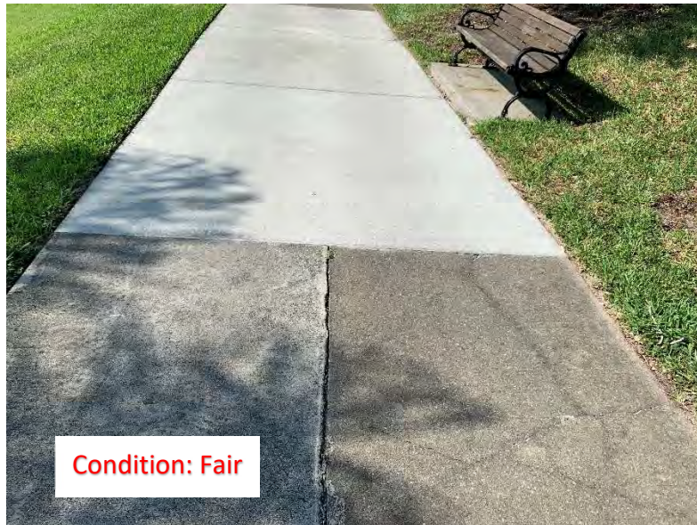
(81) Elevated Corner/Slab (1)
