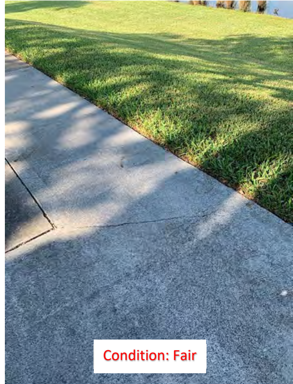
(36) Corner Cracks
