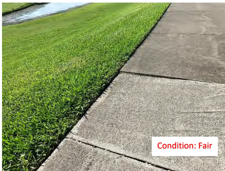
(81) Elevated Corner/Slab (2)
