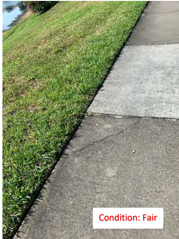
(87) Corner Cracks (2)
