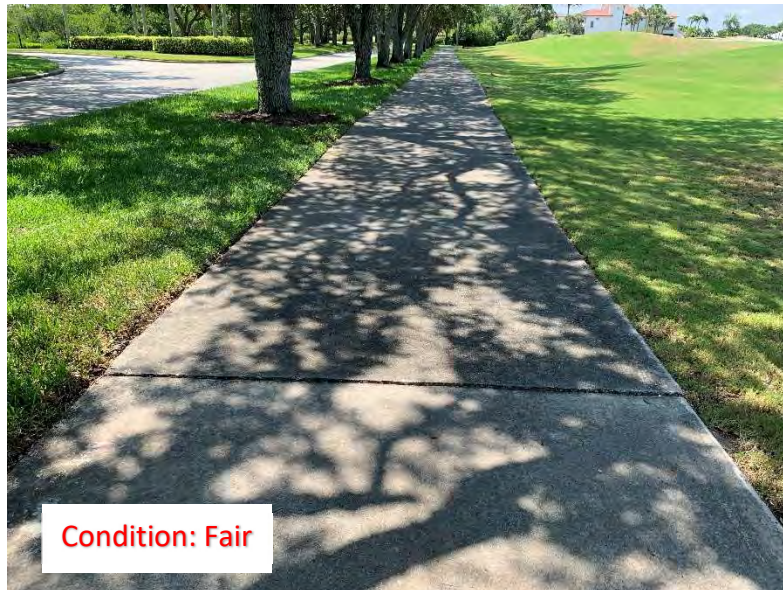
(130) Elevated Corner/Slab
