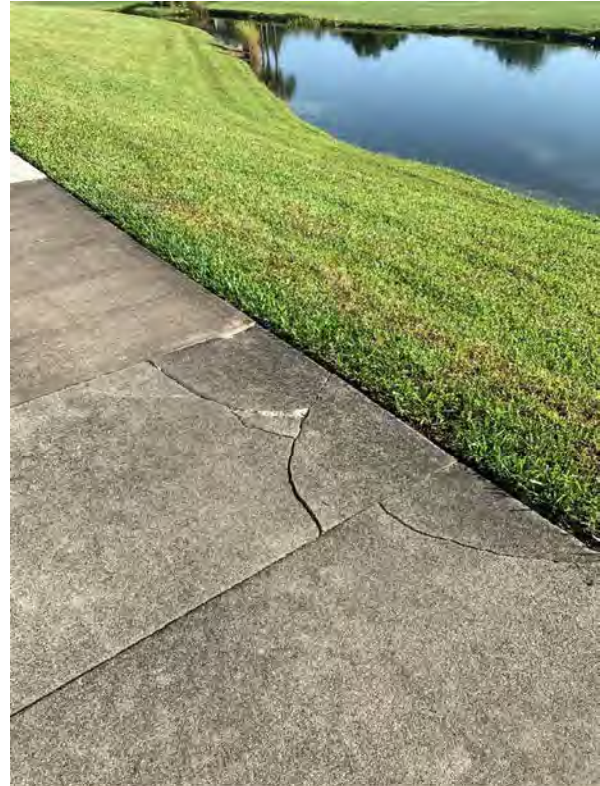
(9) Side Cracks
