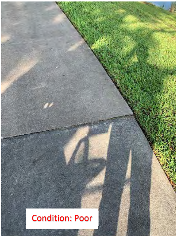
(28) Elevated Corner/Slab
