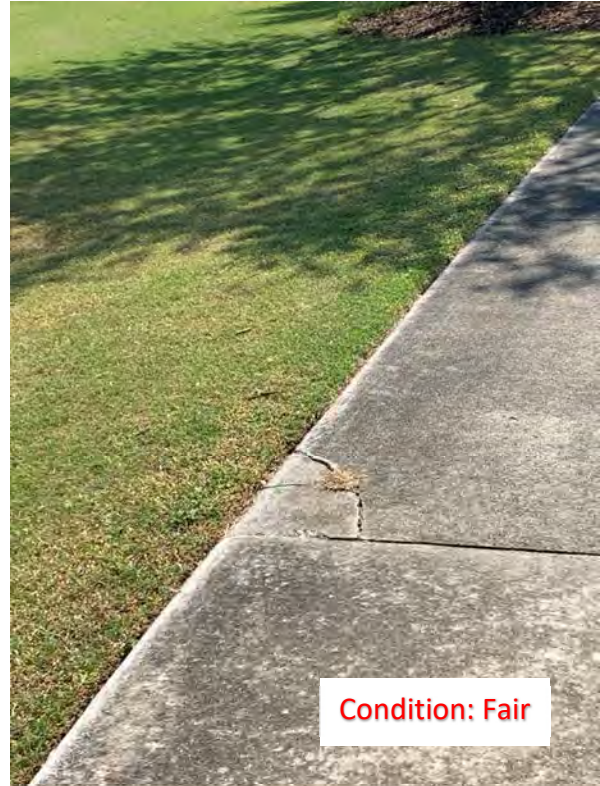
(114) Corner Cracks (3)
