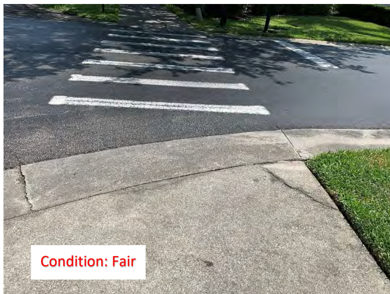
(148) Corner Cracks (1)
