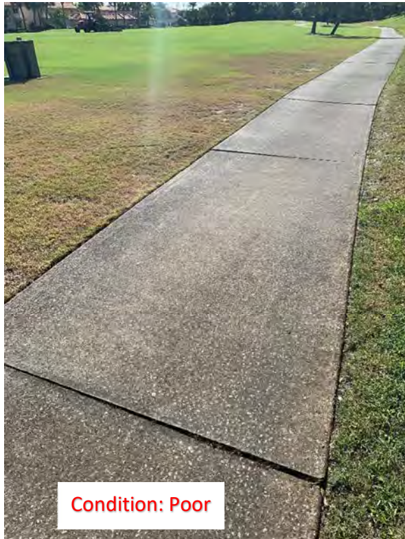
(54) Elevated Corner/Slab
