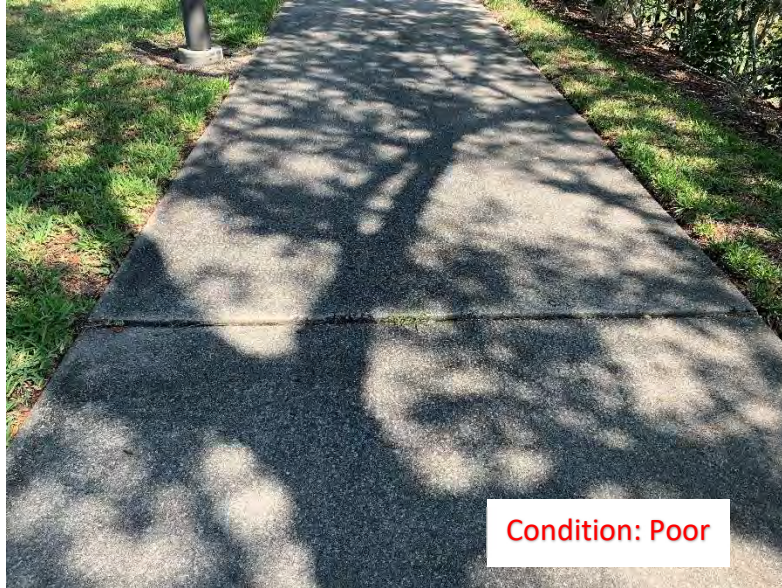
(106) Elevated Corner/Slab
