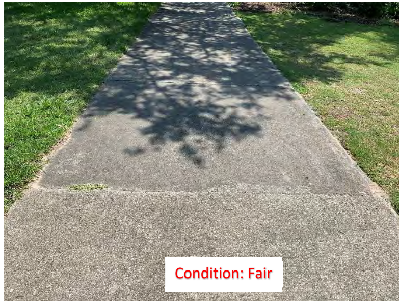
(121) Center Cracks (1)
