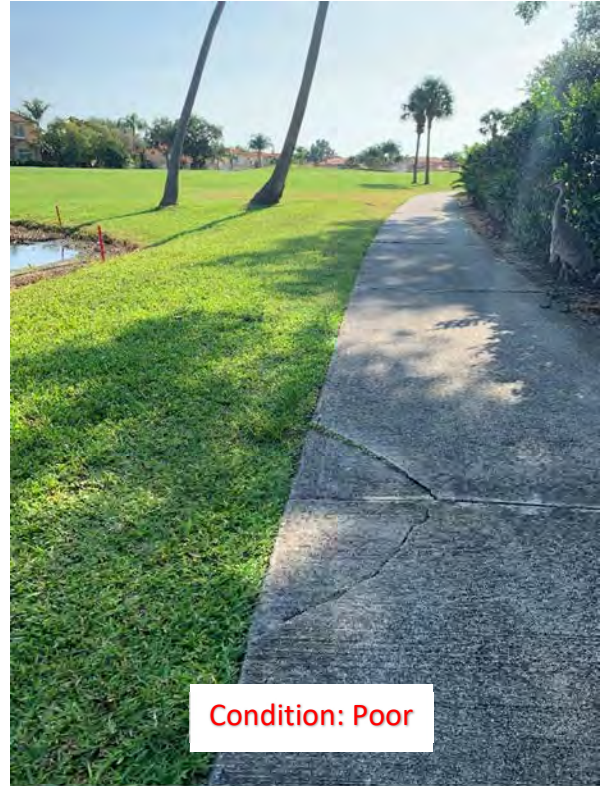
(46) Corner Cracks
