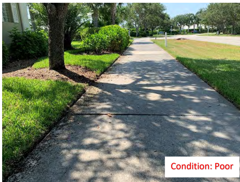
(118) Corner Cracks
