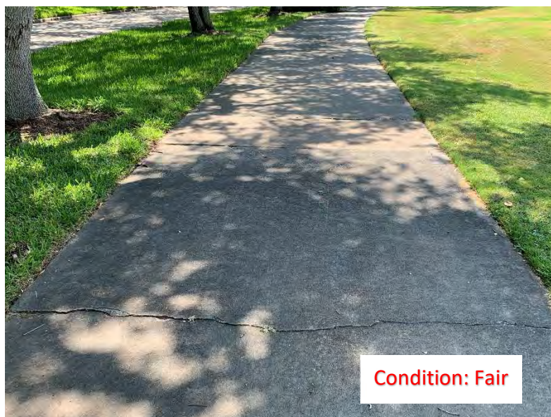
(126) Center Cracks (1)
