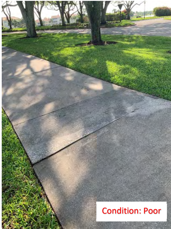
(30) Elevated Corner/Slab
