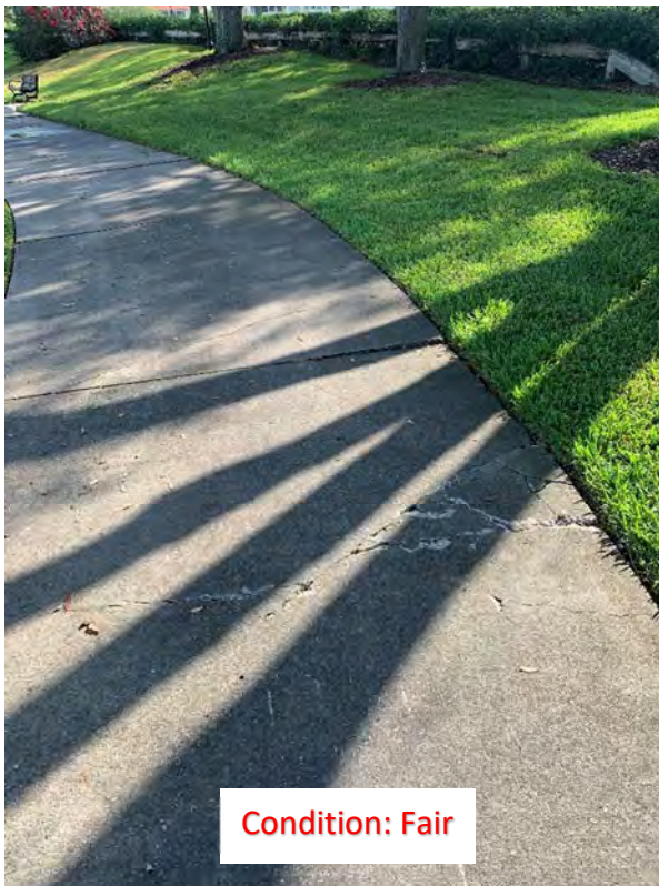
(32) Elevated Corner, Corner and Center Cracks (1 and 2)
