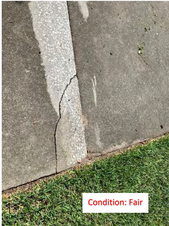
(89) Corner Crack
