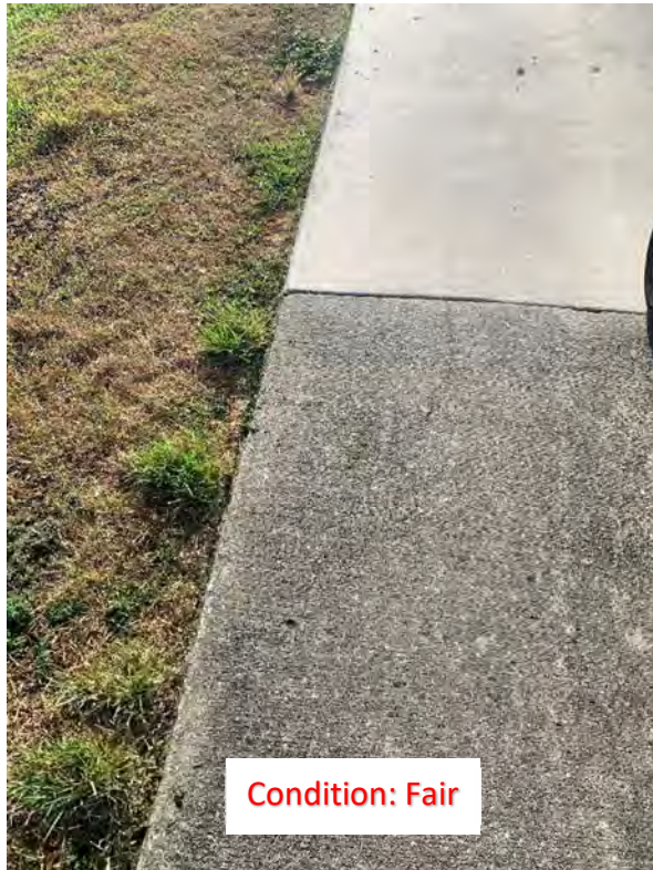
(4) Corner Cracks (2)
