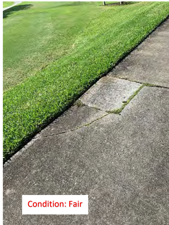
(79) Corner Crack
