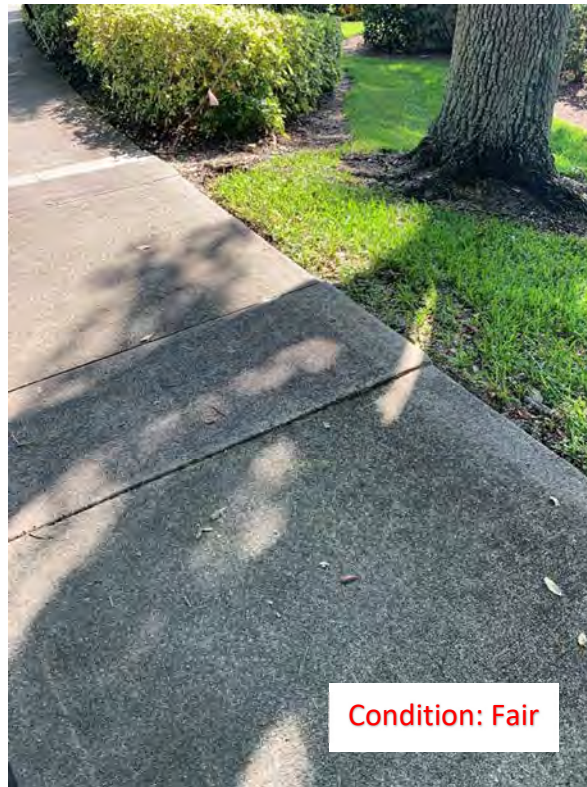
(76) Elevated Corner/Slab
