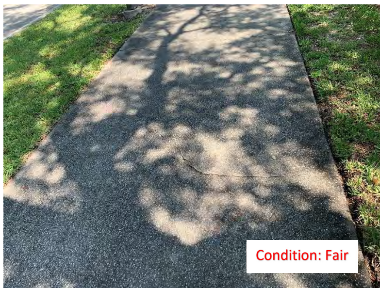
(103) Corner Cracks (2)
