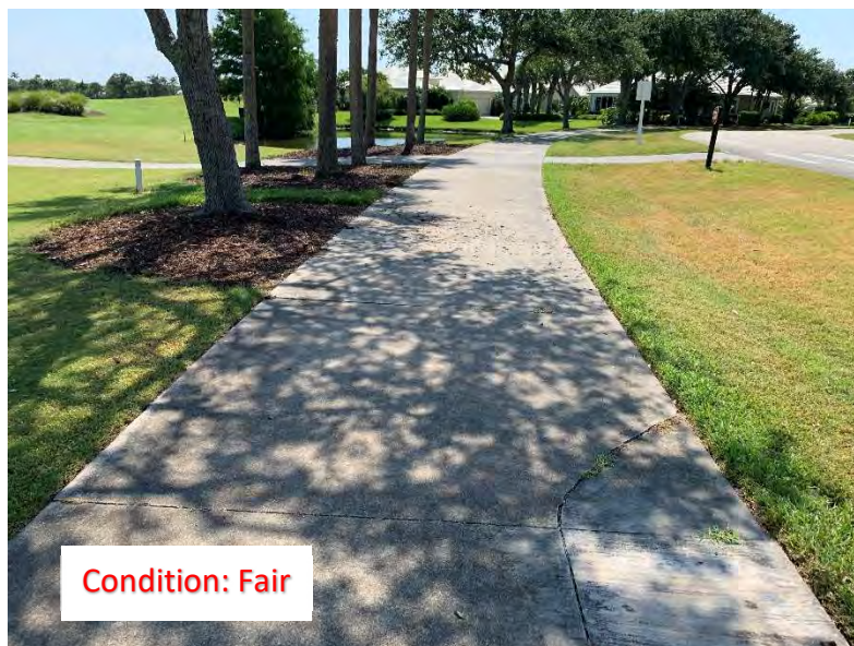
(114) Corner Cracks (4)
