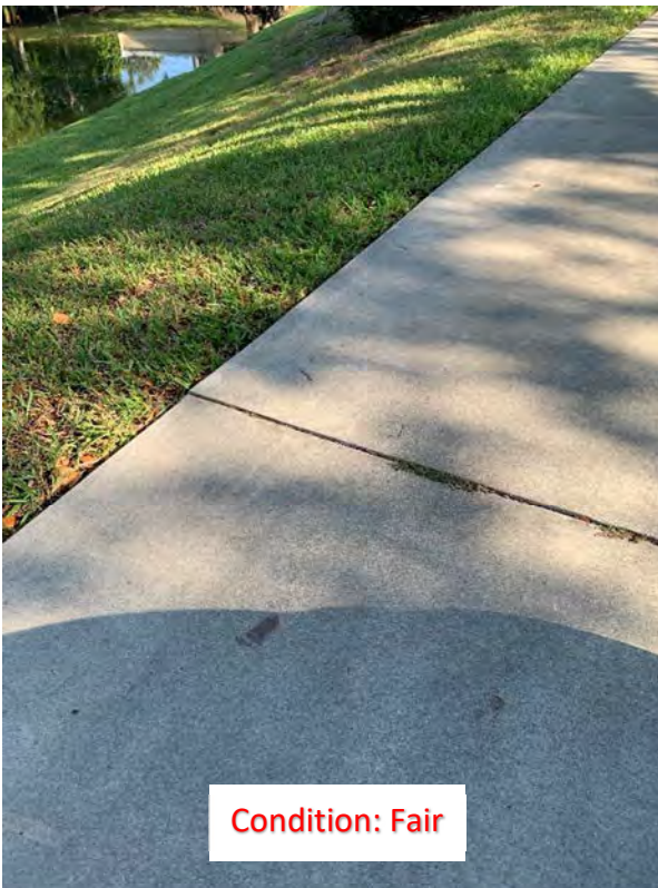
(40) Elevated Corner/Slab (2)
