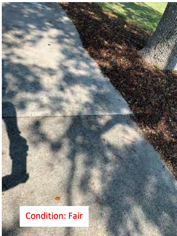
(113) Corner Crack
