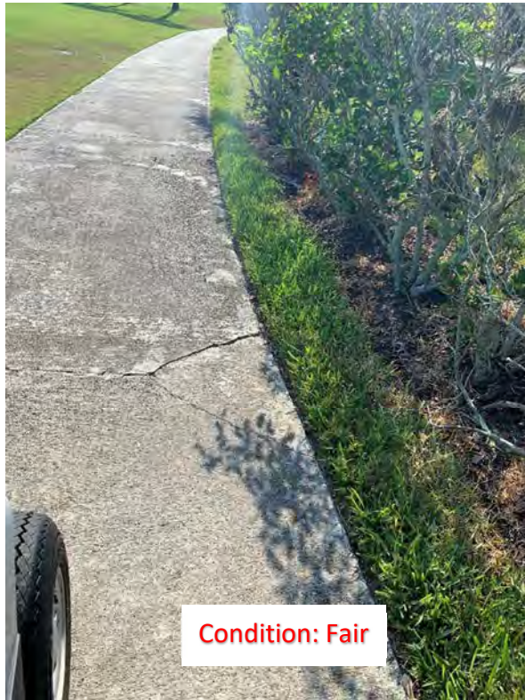
(49) Corner Cracks
