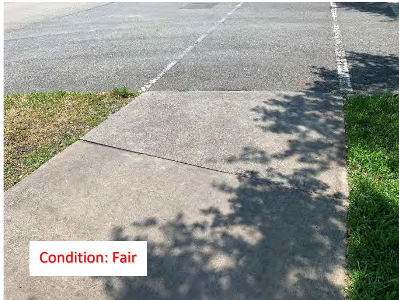
(141) Elevated Corner/Slab
