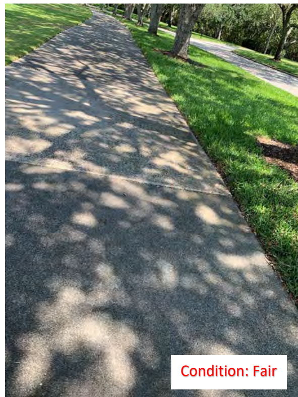
(134) Elevated Corner/Slab
