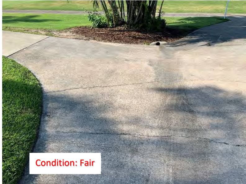
(61) Center Cracks (2)
