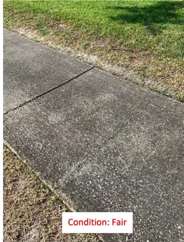
(55) Elevated Corner/Slab and Center
