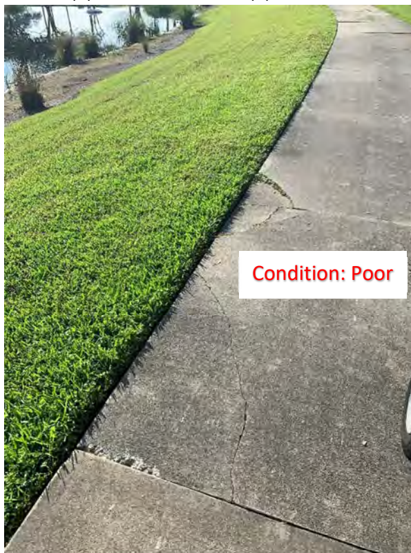
(10) Corner Cracks
