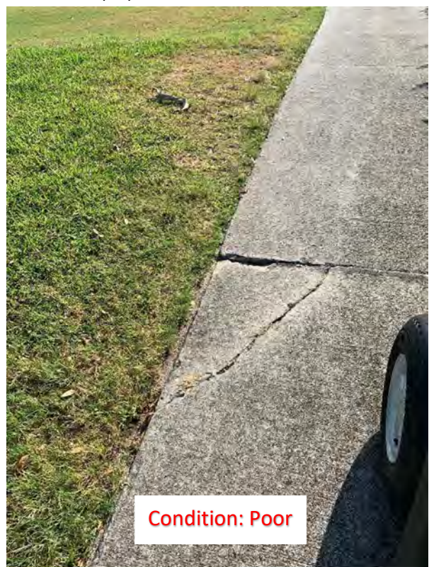
(48) Corner Crack
