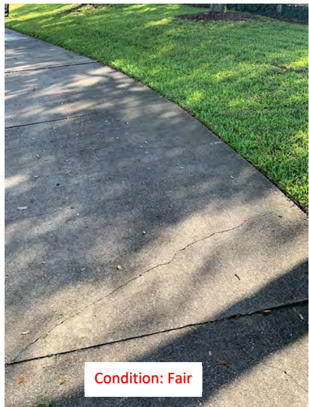
(32) Elevated Corner, Corner and Center Cracks (1 and 2)
