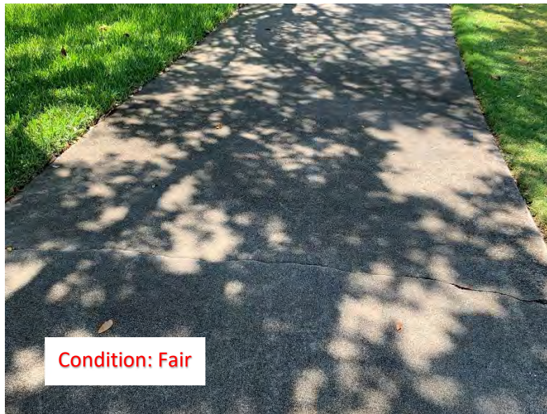
(128) Center Cracks (2)
