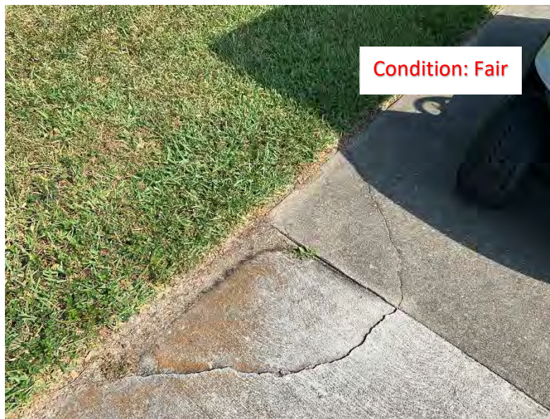
(87) Corner Cracks (3)
