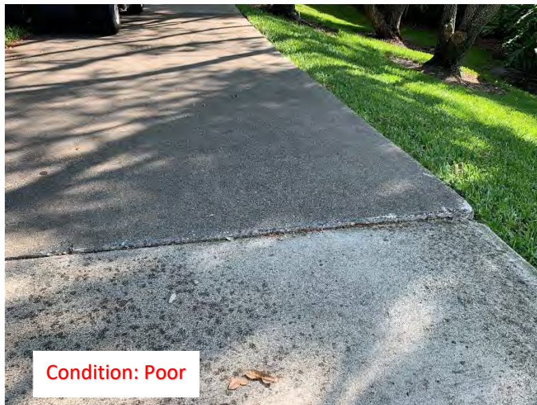
(78) Elevated Corner/Slab
