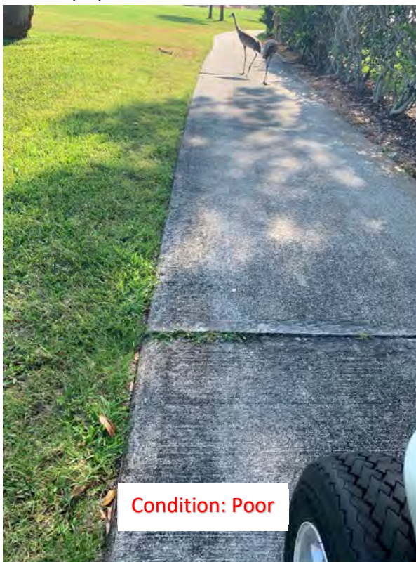
(47) Elevated Corner/Slab
