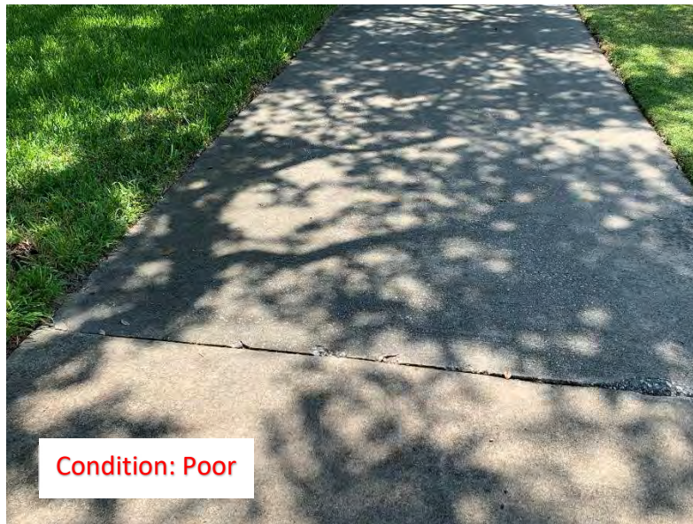
(126) Center Cracks (2)
