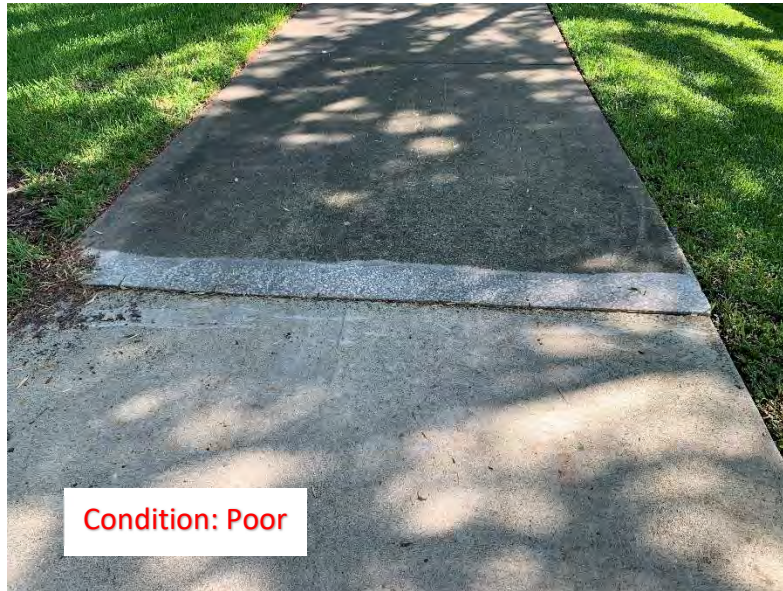
(77) Elevated Corner/Slab
