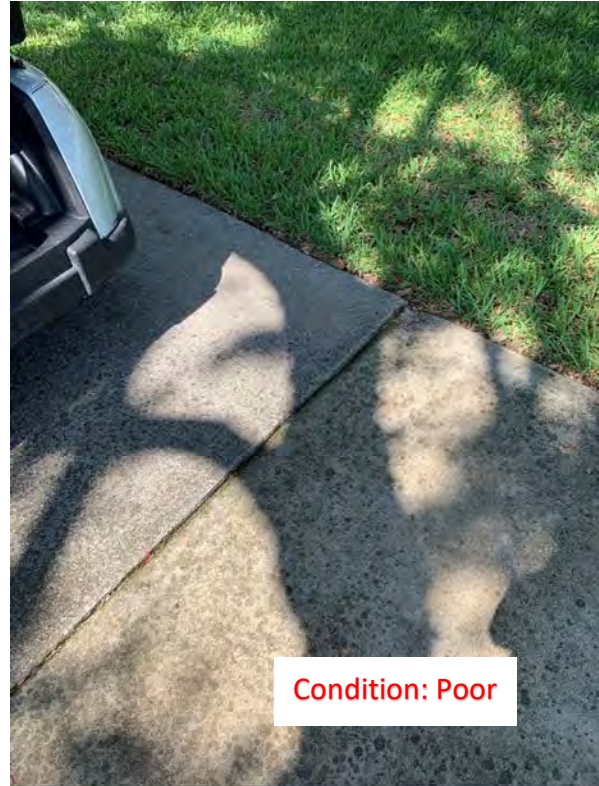
(93) Elevated Corner/Slab
