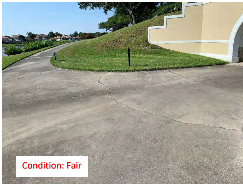
(83) Center Cracks
