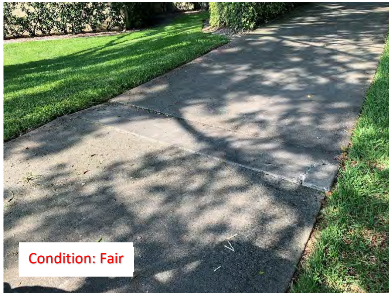
(73) Elevated Corner/Slab (2)
