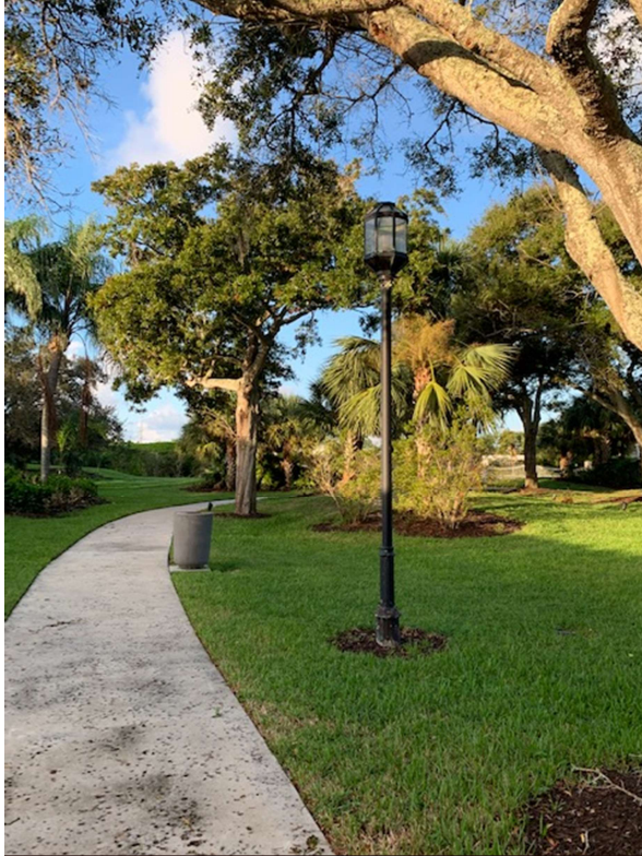
(11) Light Pole Off/Not Working
