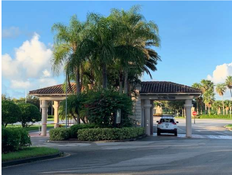
(9) Gate House Entry Light Off/Not Working
