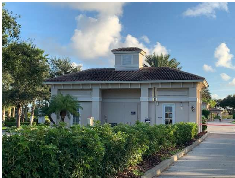
(10) Gate House Entry Small Lights Off/Not Working
