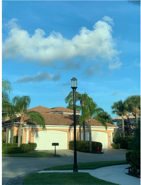
(6) Light Pole Off/Not Working
