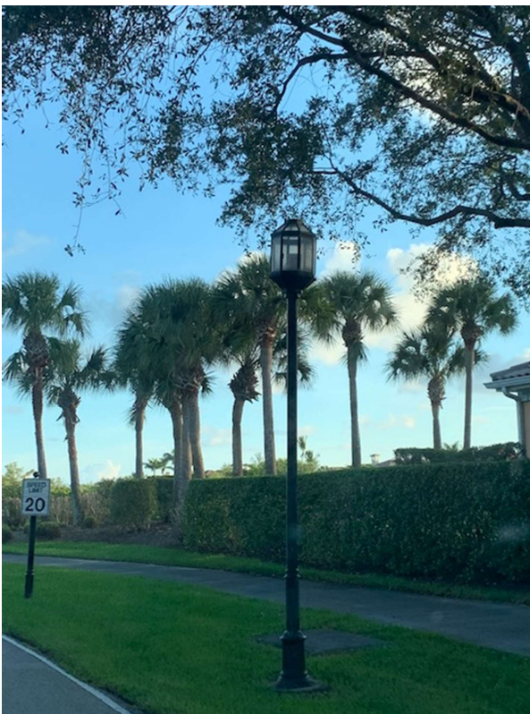
(3) Light Pole Off/Not Working
