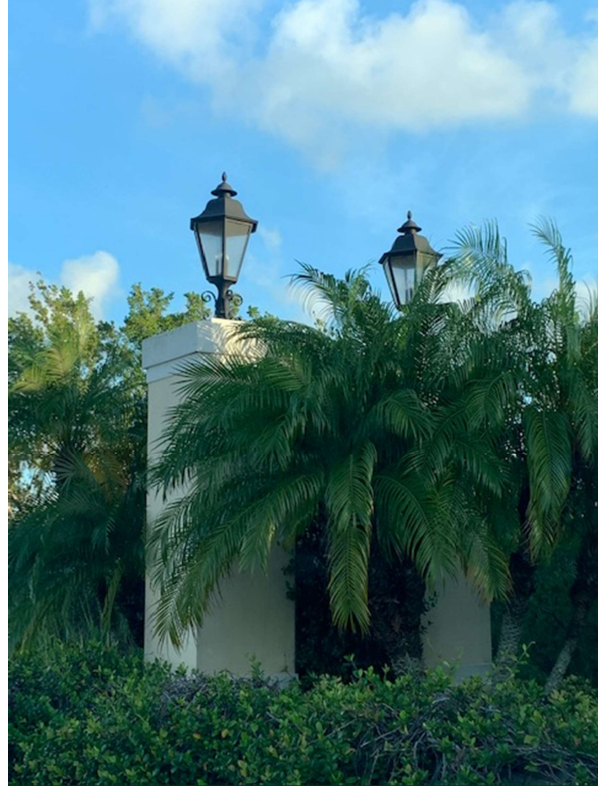
(2) Two Lights on Pillar Not Working-Lagoon Side
