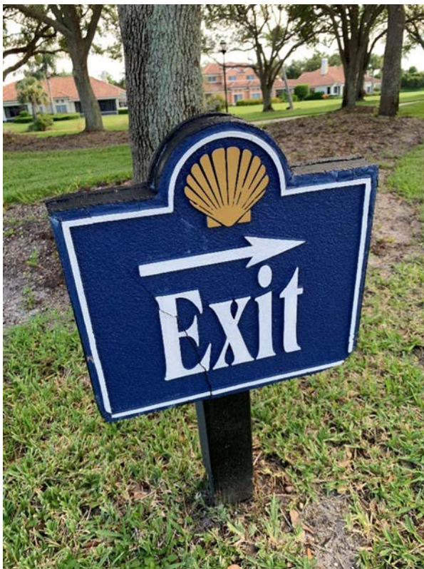
(2) Post Decay/Cracked Sign (1)
