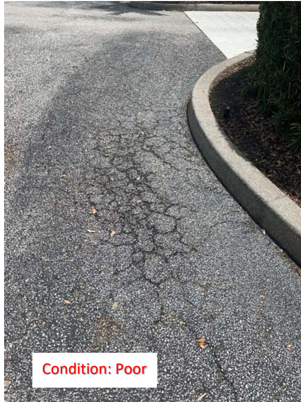
(40) Cracked Asphalt
