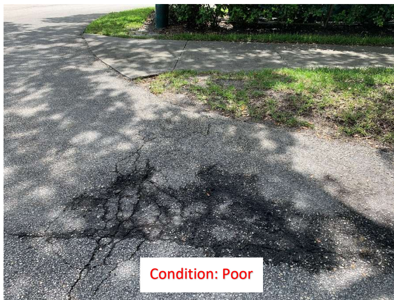
(15) Significant Cracking
