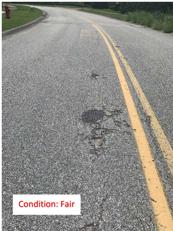
(28) Cracked Asphalt
