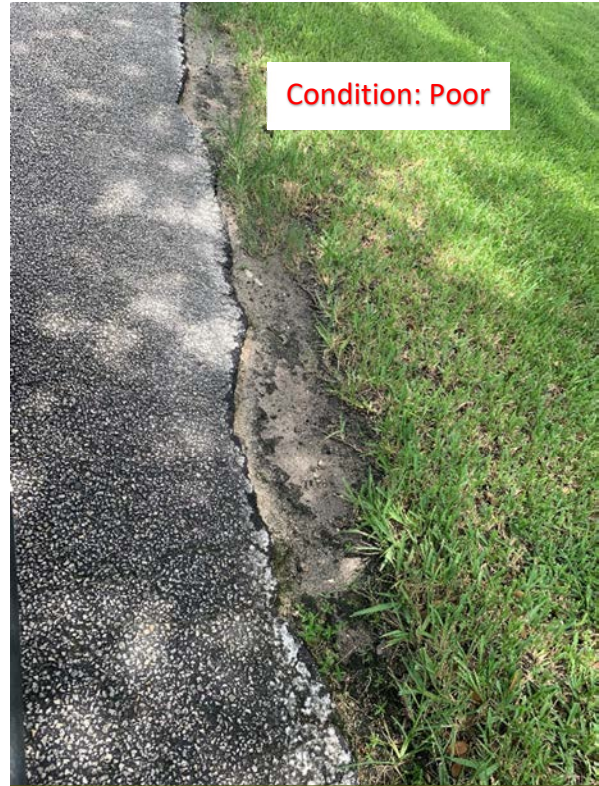
(43) Collapsed Asphalt
