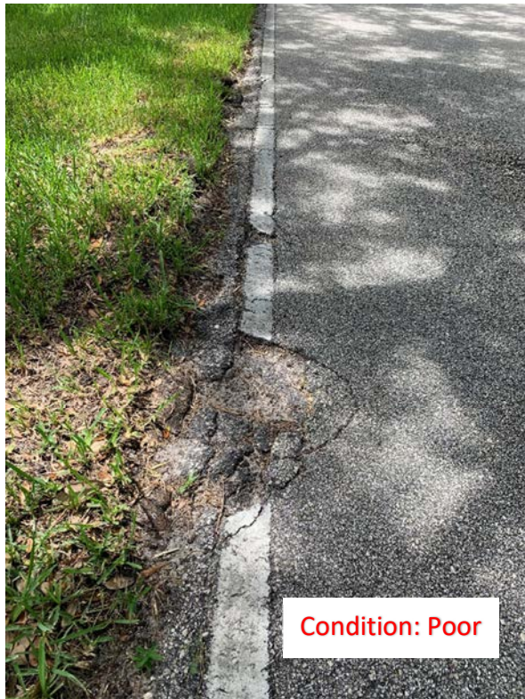
(55) Chipped Asphalt
