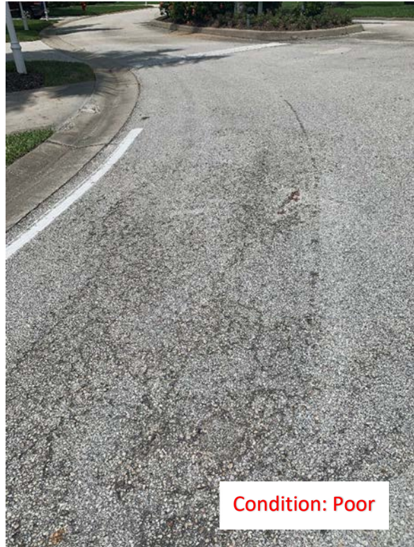
(33) Cracked Asphalt
