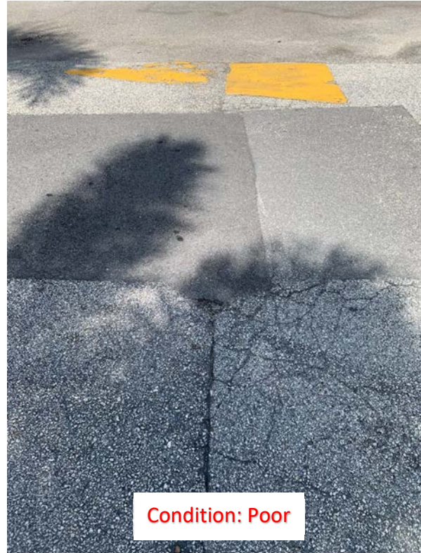
(6) Cracked Asphalt
