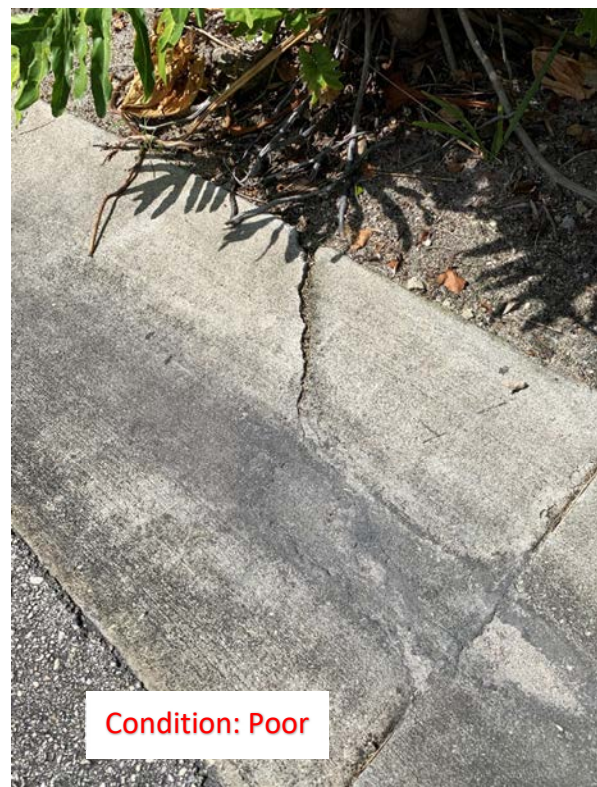
(4) Cracked Gutter
