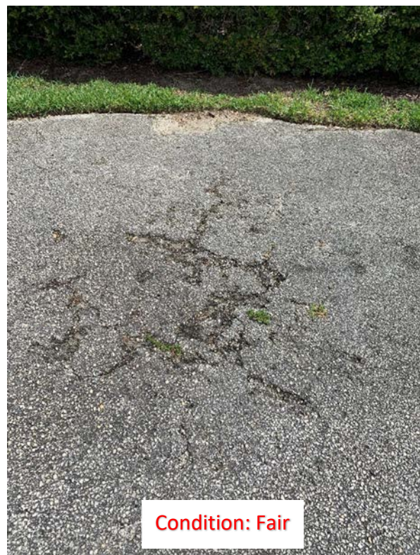
(12) Significant Cracking
