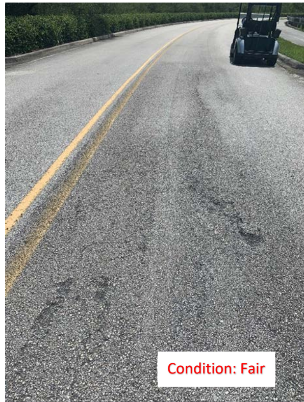
(31) Cracked Asphalt
