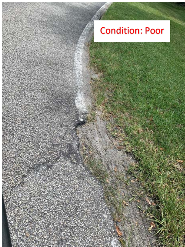
(44) Collapsed Asphalt
