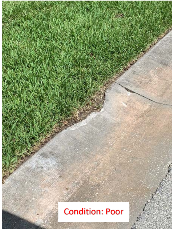
(5) Chipped Gutter
