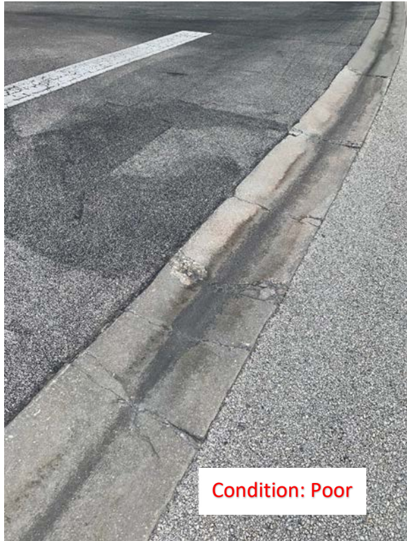
(9) Chipped Gutter
