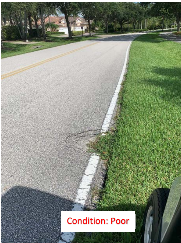
(3) Asphalt Collapse
