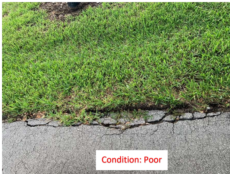
(59) Chipped Asphalt
