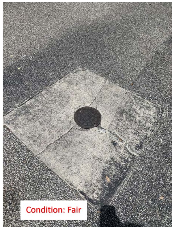
(39) Chipped Concrete
