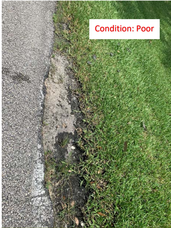
(42) Collapsed Asphalt
