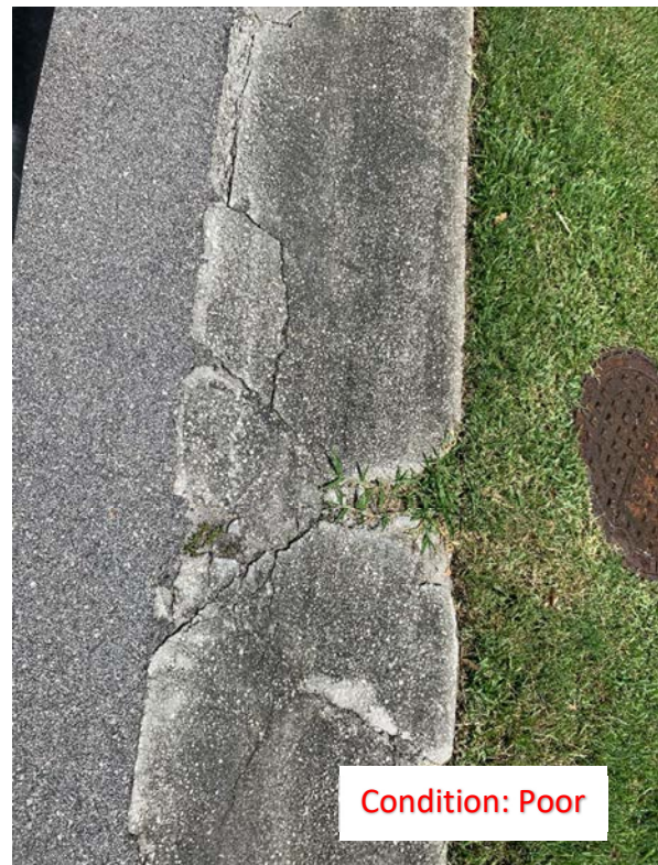
(12) Gutter Chipped/Cracked
