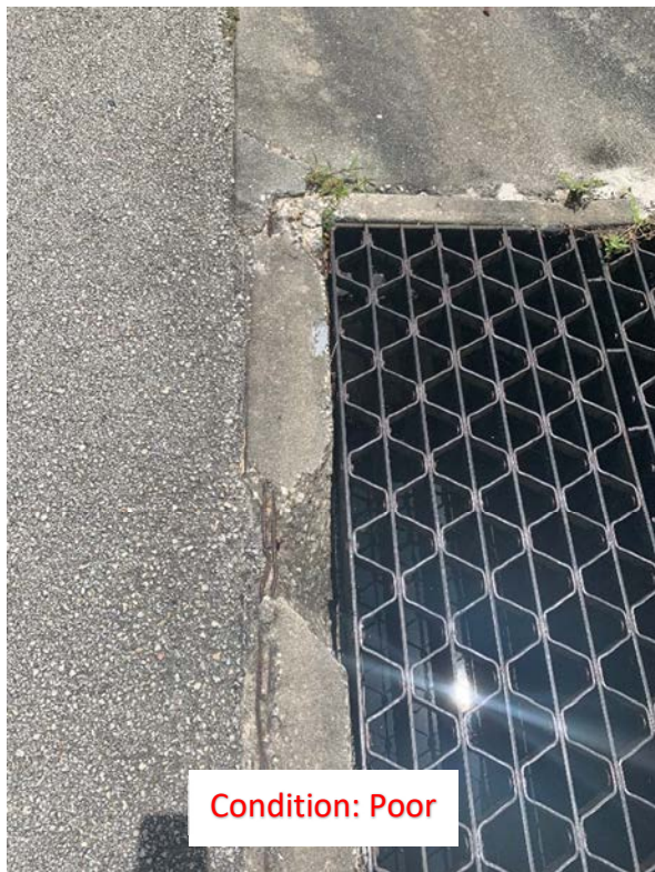
(11) Chipped Concrete
