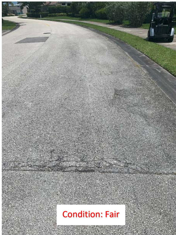
(30) Cracked Asphalt
