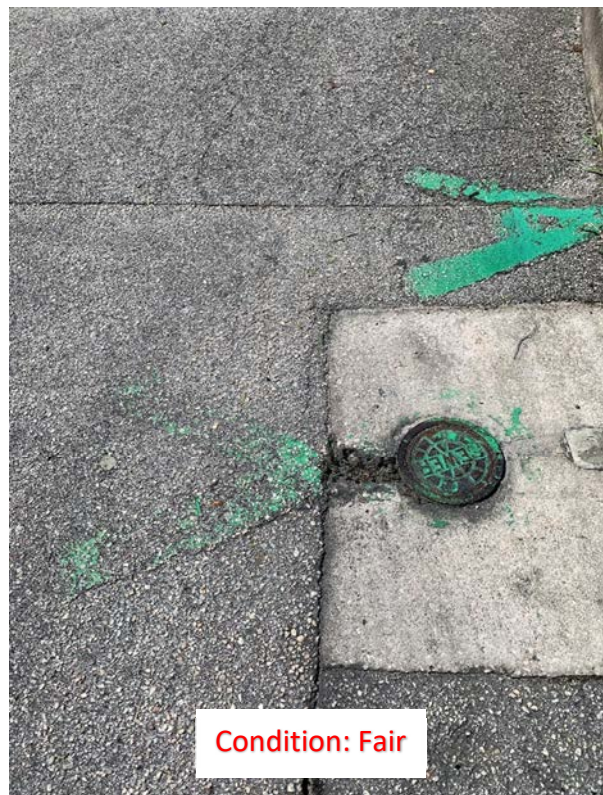
(8) Concrete Crack
