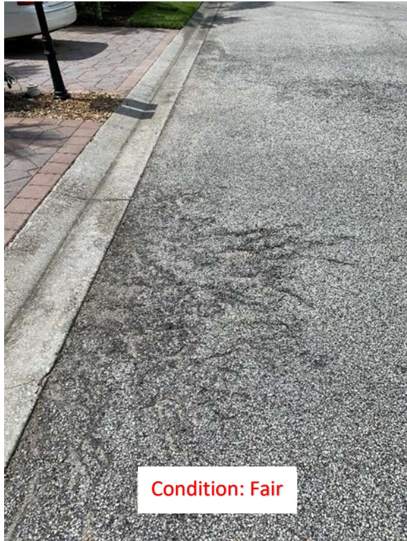
(13) Significant Cracking
