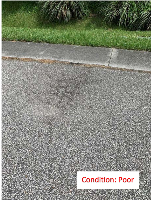
(22) Significant Cracking/Dip
