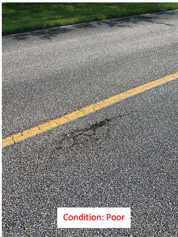
(38) Cracked Asphalt
