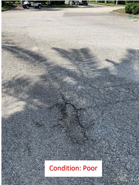
(9) Significant Cracking
