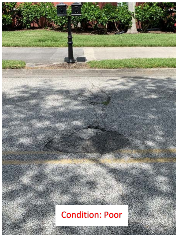
(11) Significant Cracking
