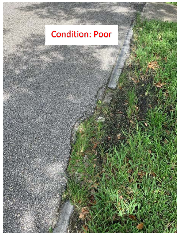
(49) Collapsed Asphalt
